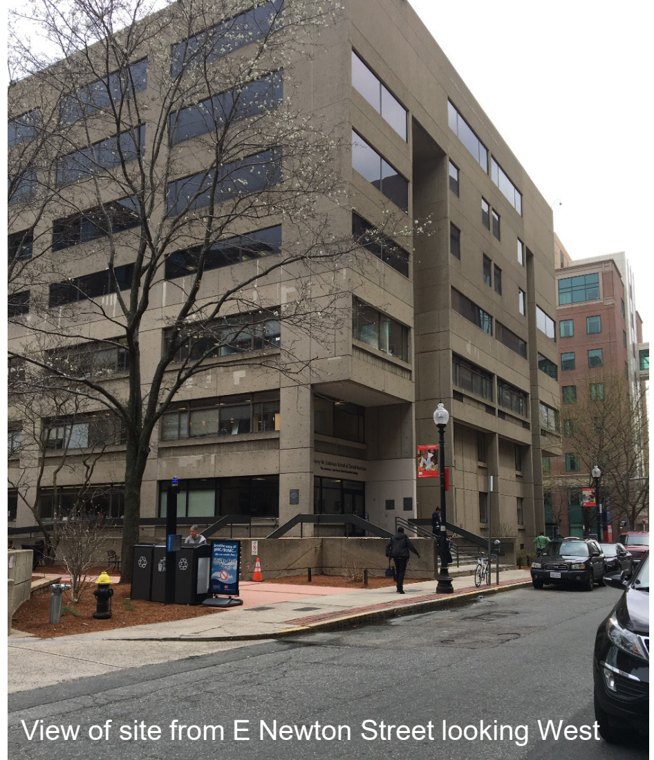
View of site from Albany & E Newton Streets
