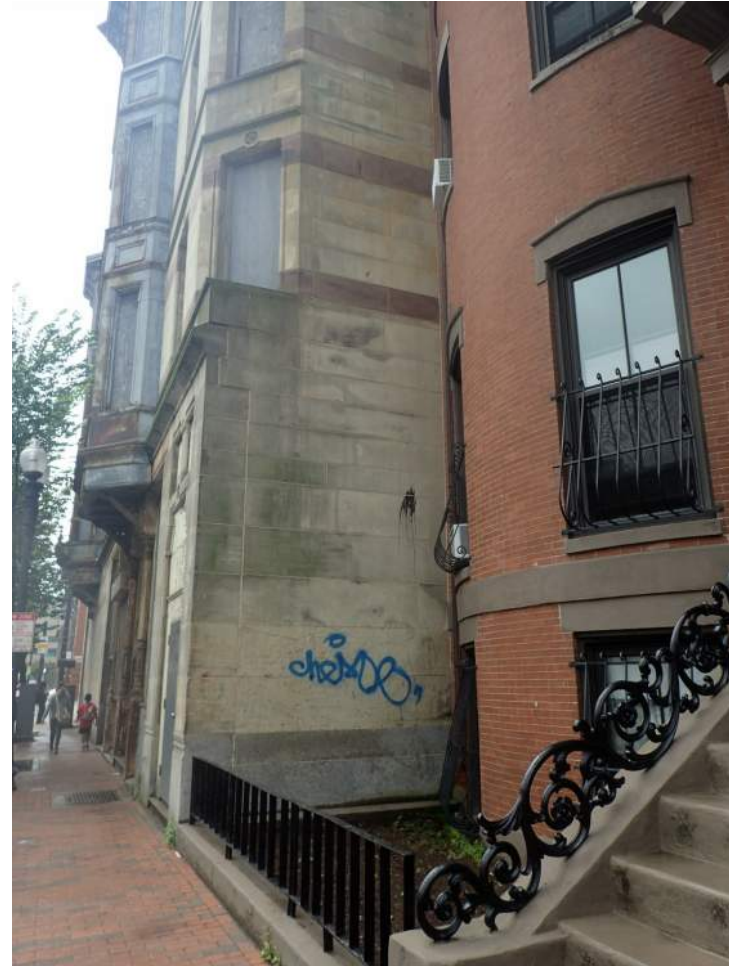
BOTTOM OF NORTH ELEVATION
