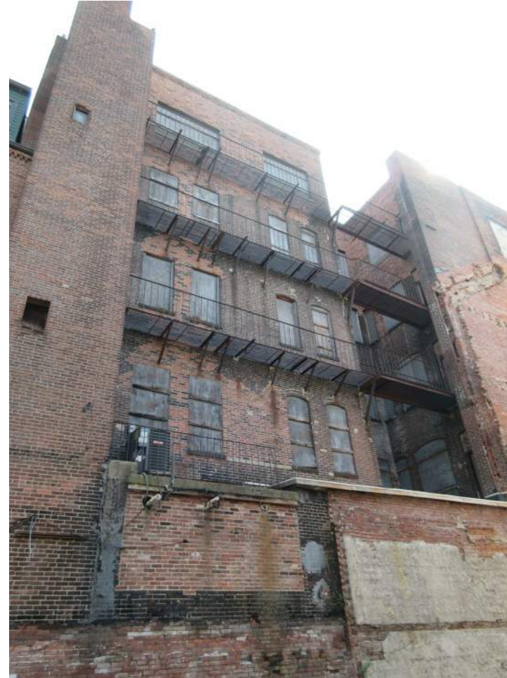
WEST ELEVATION FROM COMET PLACE
