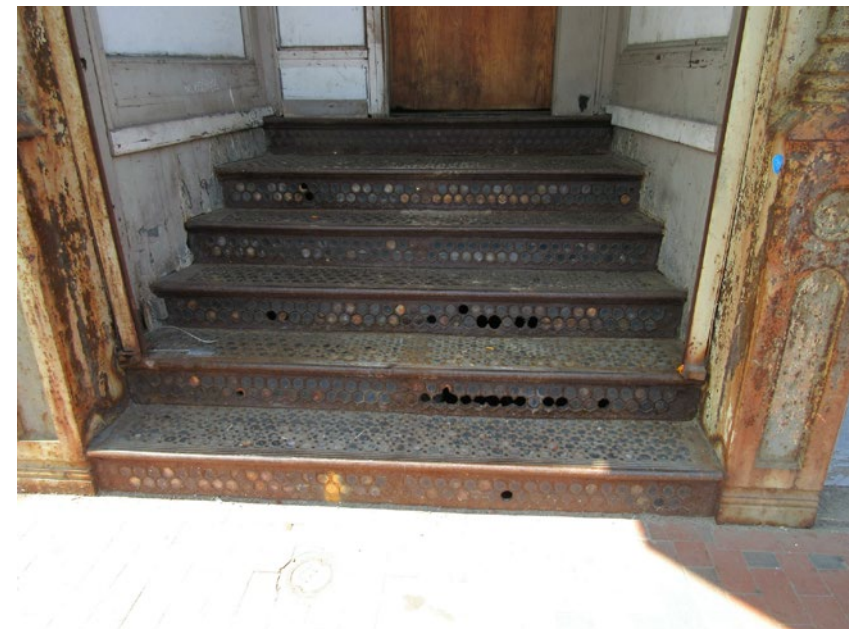
CAST IRON STAIRS WITH PRISM LIGHTS
