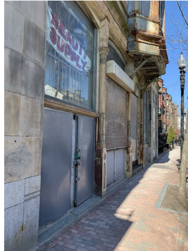
STOREFRONT AND OPENINGS AT EAST ELEVATION
