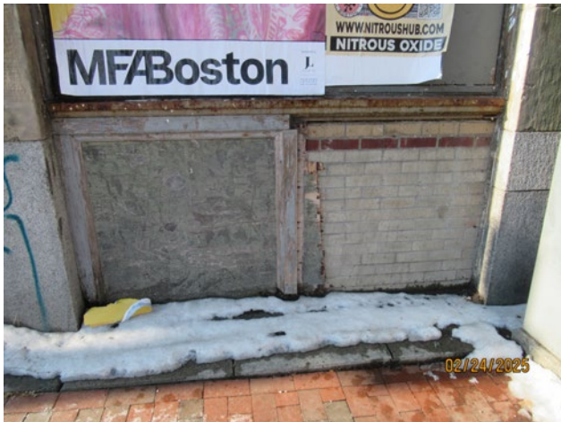
BRICK INFILL BEHIND PANEL
