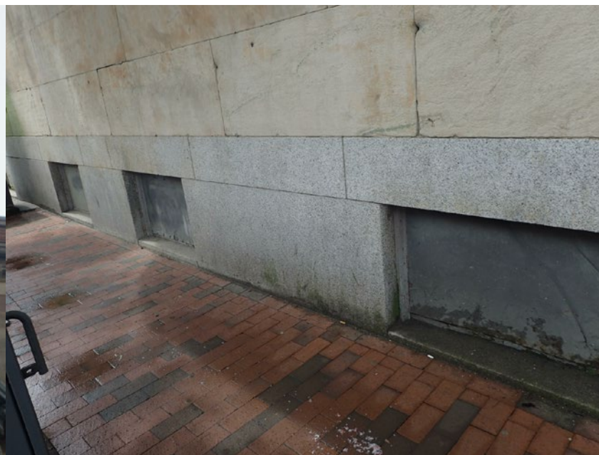
GRANITE BASE AND INFILLED BASEMENT WINDOWS AT EAST ELEVATION
