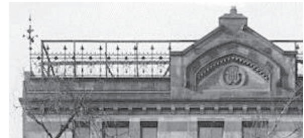
2 DETAIL OF TYPICAL NEW ROOF CRESTING AND FINIAL 3/8" = 1'-0"
