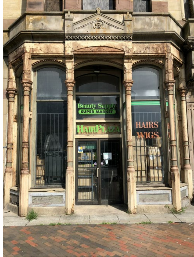
CAST IRON STOREFRONT AT SOUTH ELEVATION
