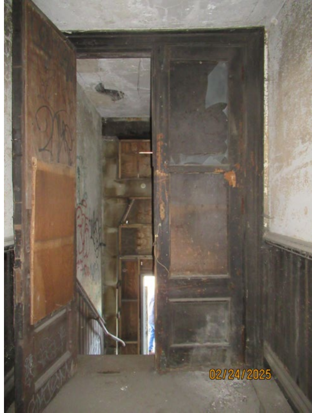
ORIGINAL DOORS AT REAR
