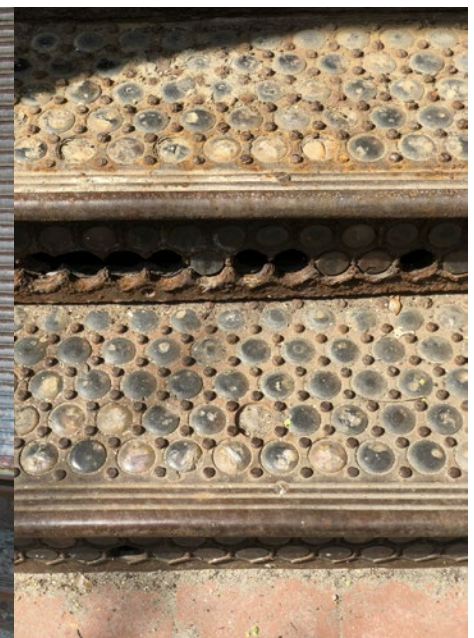
CLOSE-UP OF CAST IRON STAIR
