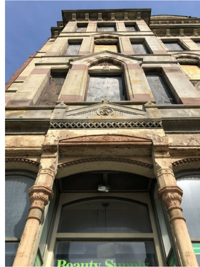
VIEW OF WEST BAY AT SOUTH ELEVATION
