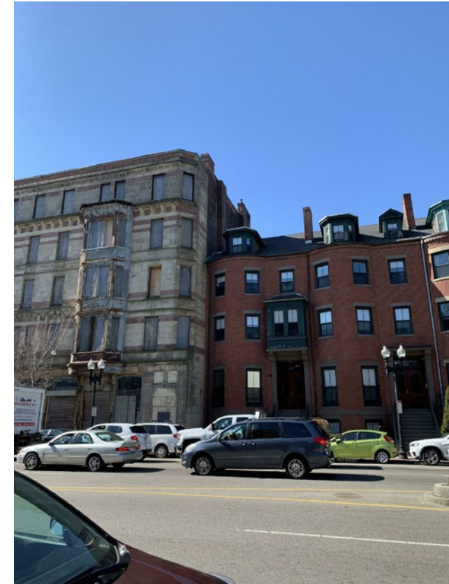
VIEW OF NORTHEAST CORNER
