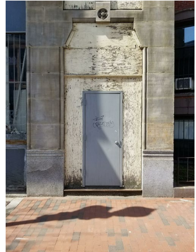
NON-ORIGINAL DOOR AND INFILL AT EAST ELEVATION
