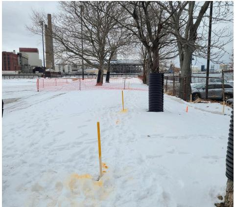
Tree protection includes both protecting the trunk from accidental contact, and protecting the earth under the dripline from being compacted if it gets driven over – using bright orange plastic fencing.
