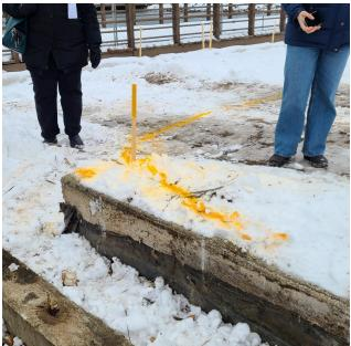
Yellow spray indicates the gas line - it turns within our site limits, which was not reflected on drawings. Site conditions frequently differ from record drawings. With a large gas line, it's clearly important to make sure to get it right.
