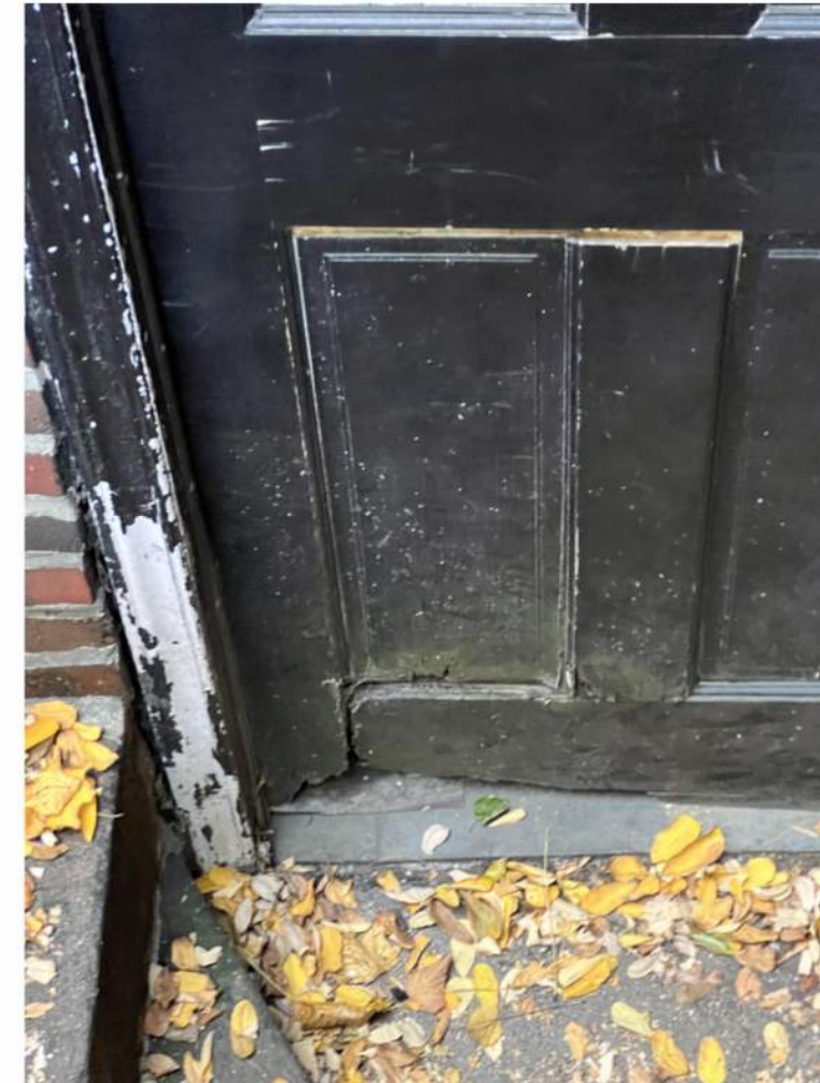
EXAMPLE OF WATER DAMAGED SIDE DOOR
