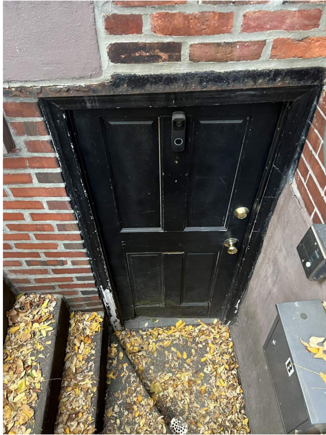
VIEW OF SIDE DOOR GARDEN LEVEL ENTRY
