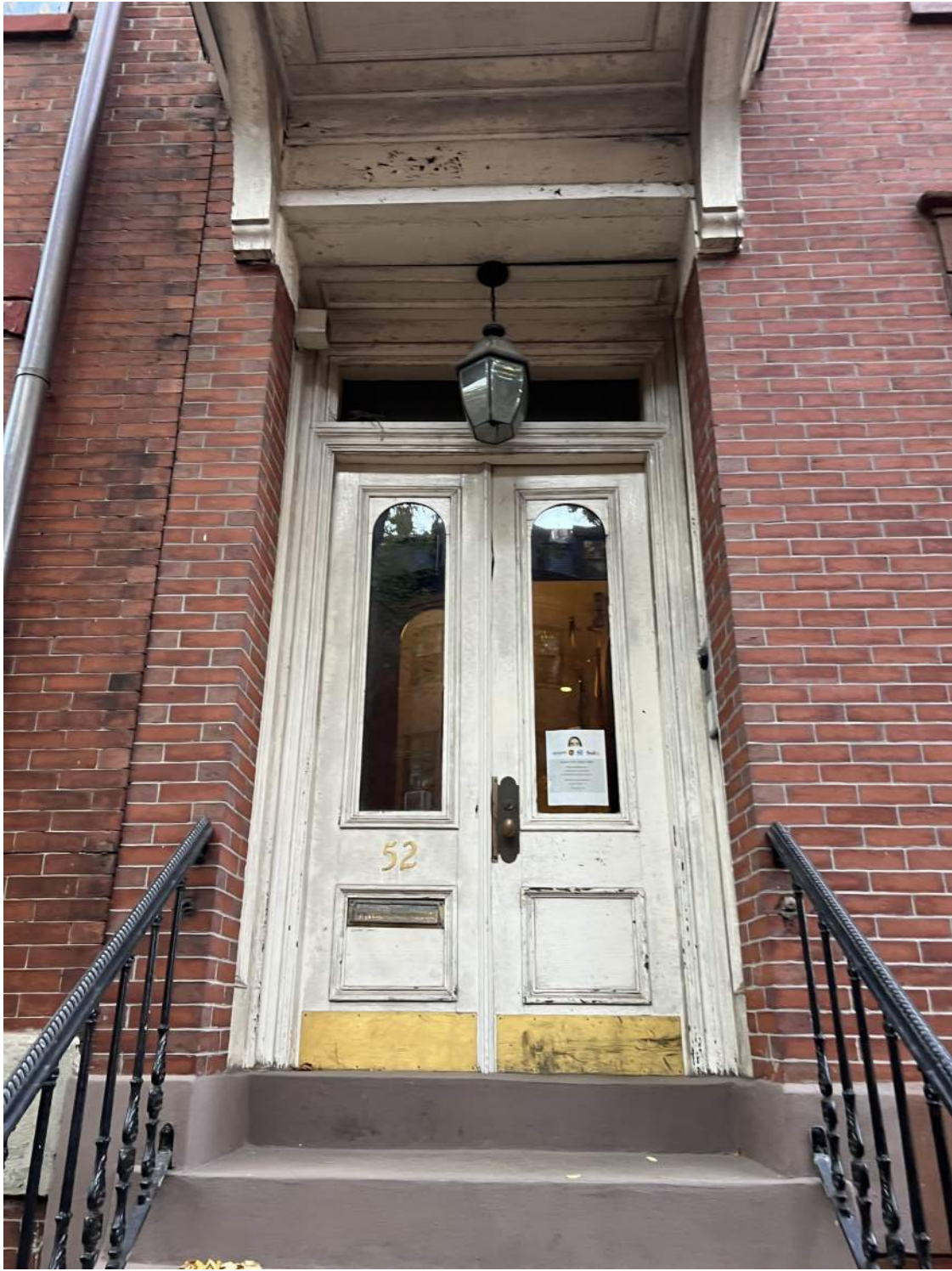
VIEW OF FRONT DOOR ENTRYWAY
