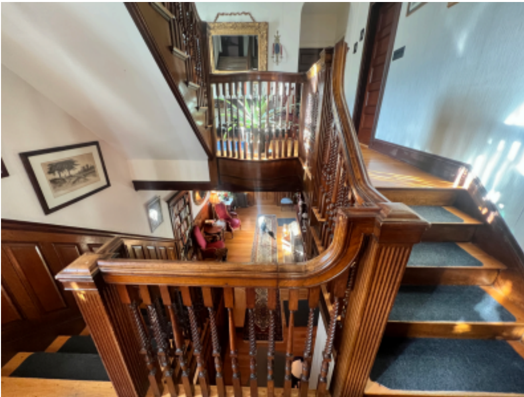
Figure 13. Looking south down grand stairs from second floor to first floor. Photograph taken in 2024.
