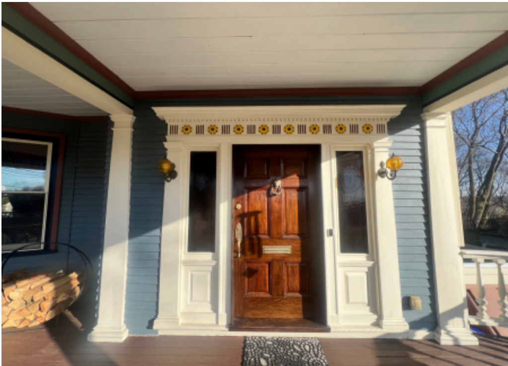
Figure 5. South-facing front entrance. Photograph taken in 2024.
