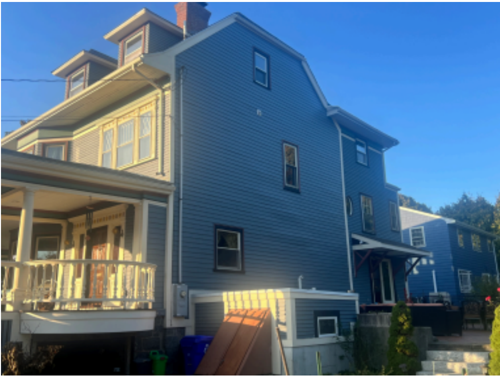
Figure 4. East facade where the house was cut. Photograph taken 2024.
