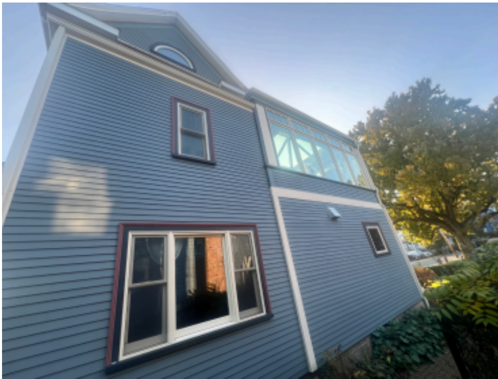
Figure 3. North façade facing 44 Maynard Street. Photograph taken 2024.
