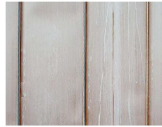
PHOTOGRAPH: EXISTING COPPER STANDING METAL SEAM SIDING
