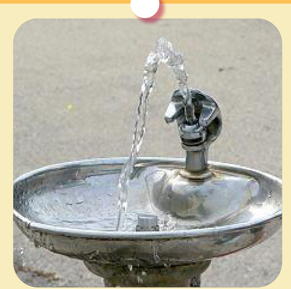
DRINKING FOUNTAIN 飲水設施
