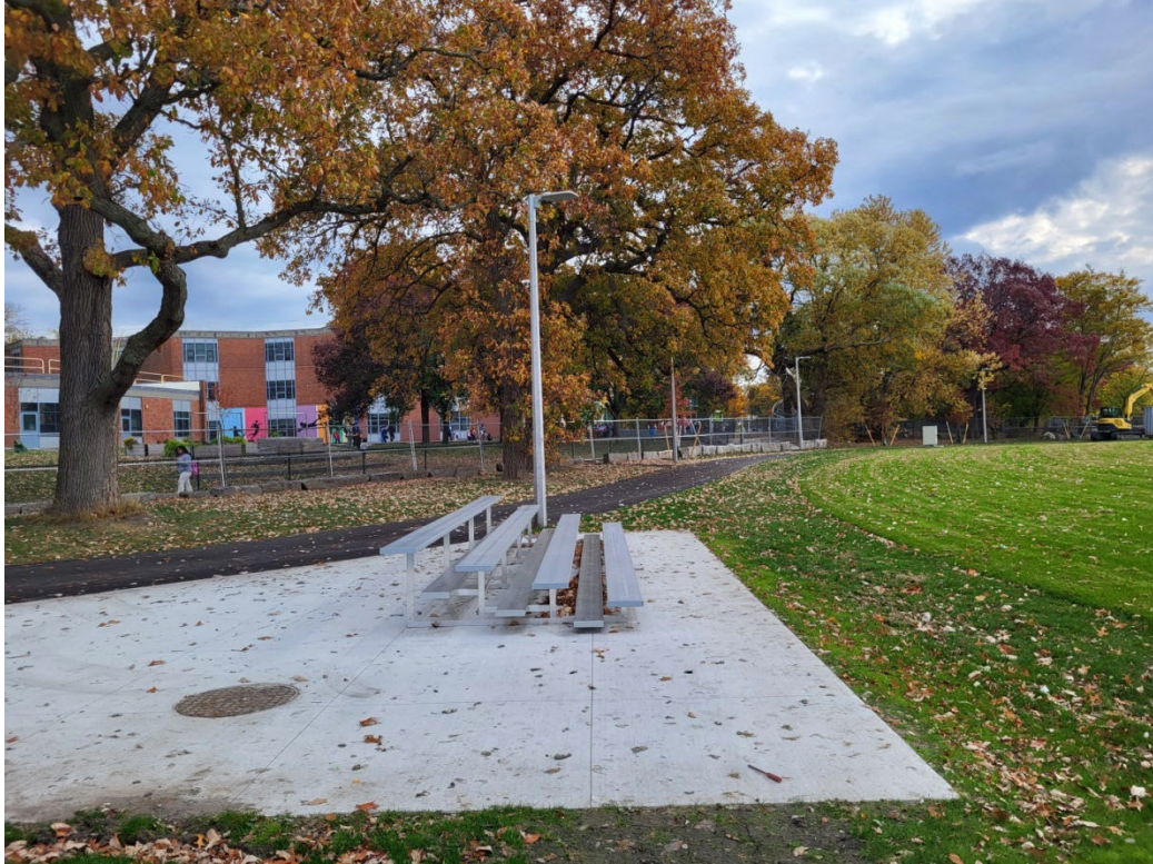
Concrete paving at bleacher location at the practice field.
