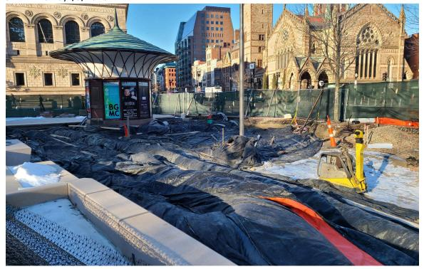
In order to excavate down and install gravel below the pervious paver area, the contractor has covered this with tarp and is heating it.
