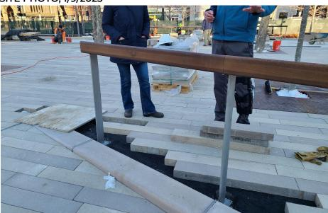
Lean rail sections were manufactured 1/8" longer than called for. If it were a short stretch of rail, this wouldn't matter much, but over 40' this difference adds up.
