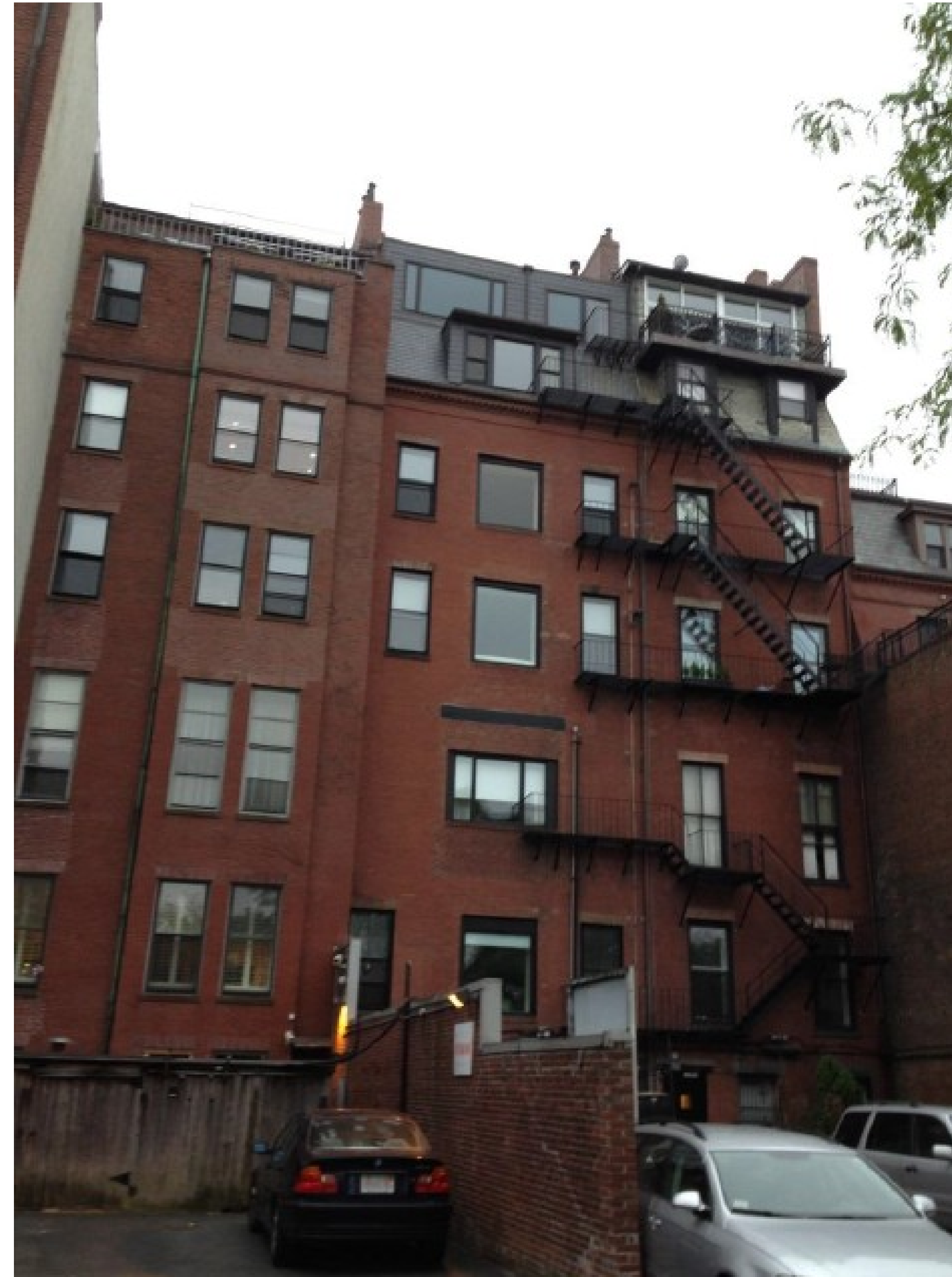
VIEW FROM REAR ALLEY
