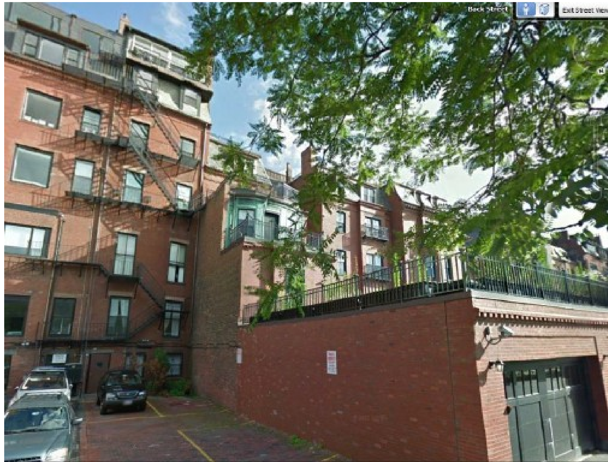
VIEW FROM REAR ALLEY
