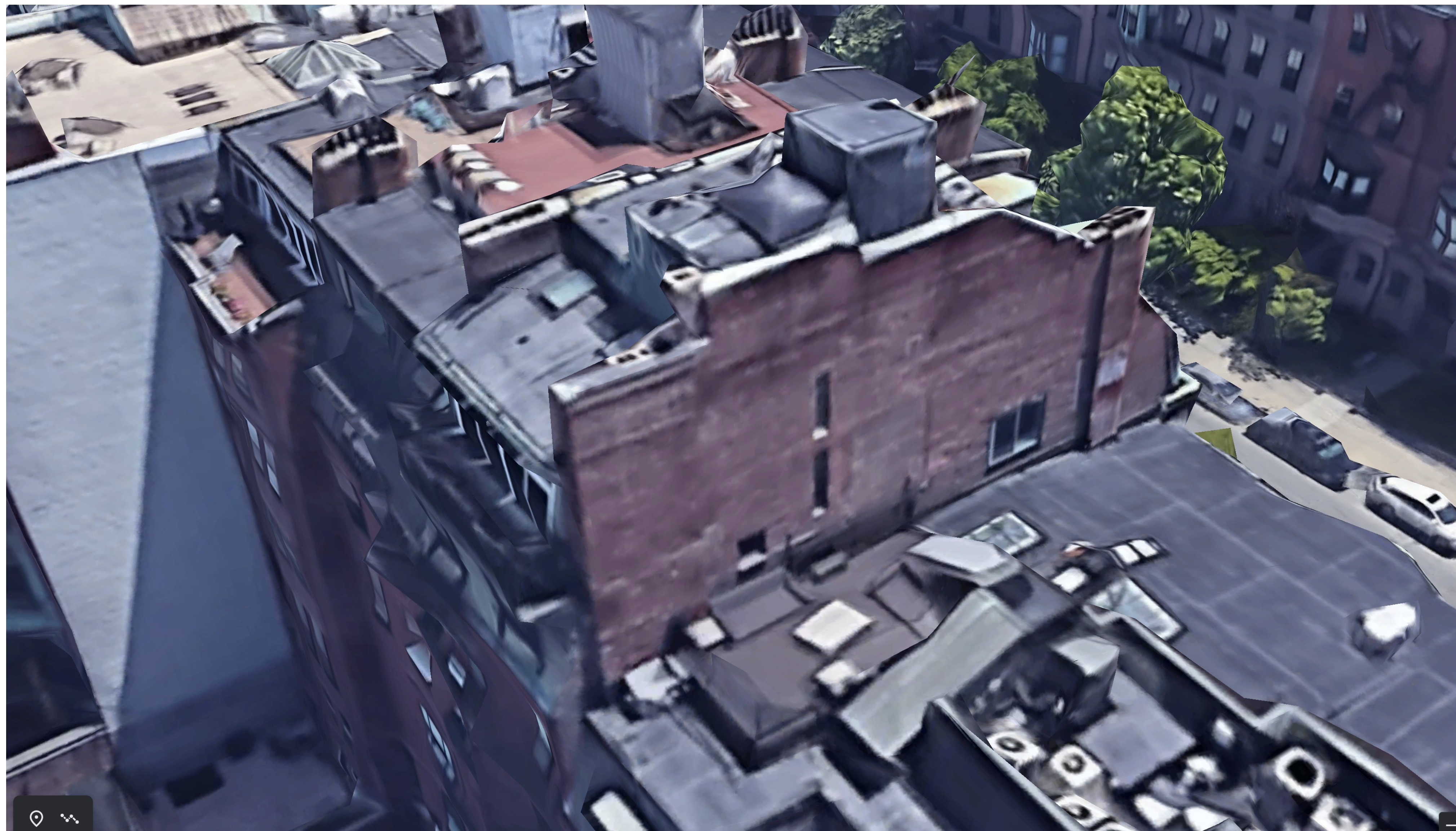
AERIAL VIEW LOOKING NORTH-
