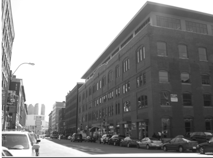
Fig. 8. American Railway Express Co. stables, 343 Congress Street, built 1888 (#42)
