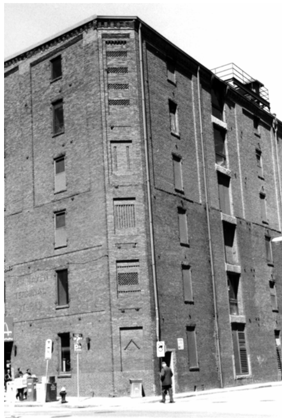
Fig. 2. Atlas Stores, 316 Congress Street, with its Panel Brick decoration in the chamfer of the Congress Street façade.
