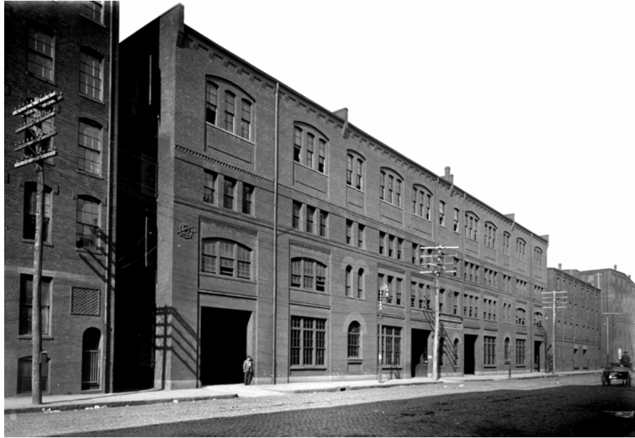
Fig. 3. Romanesque Revival, American Railway Express Building, 343 Congress Street, photographed c. 1900 (fifth floor added later).
