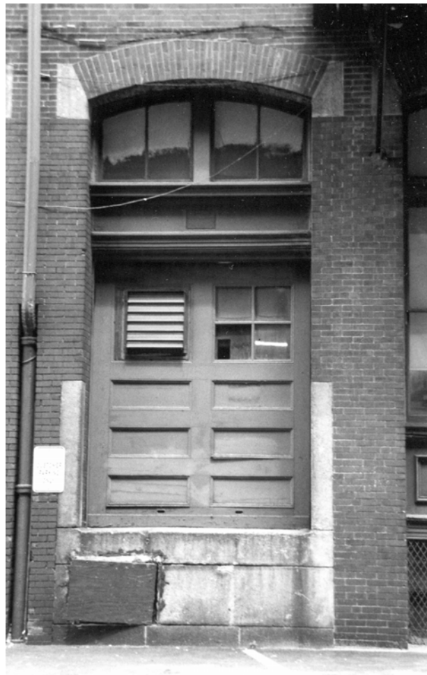
Fig. 24. Loading door with original wooden door, 311-319 Summer Street.
