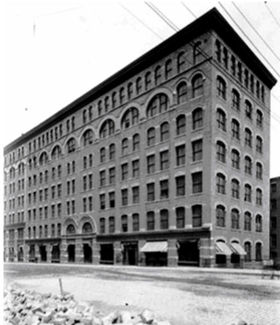
Fig. 6. Summer Street wool warehouse of Jeremiah Williams & Co. in high-style Classical, 292-302 Summer Street, photo c. 1900.
