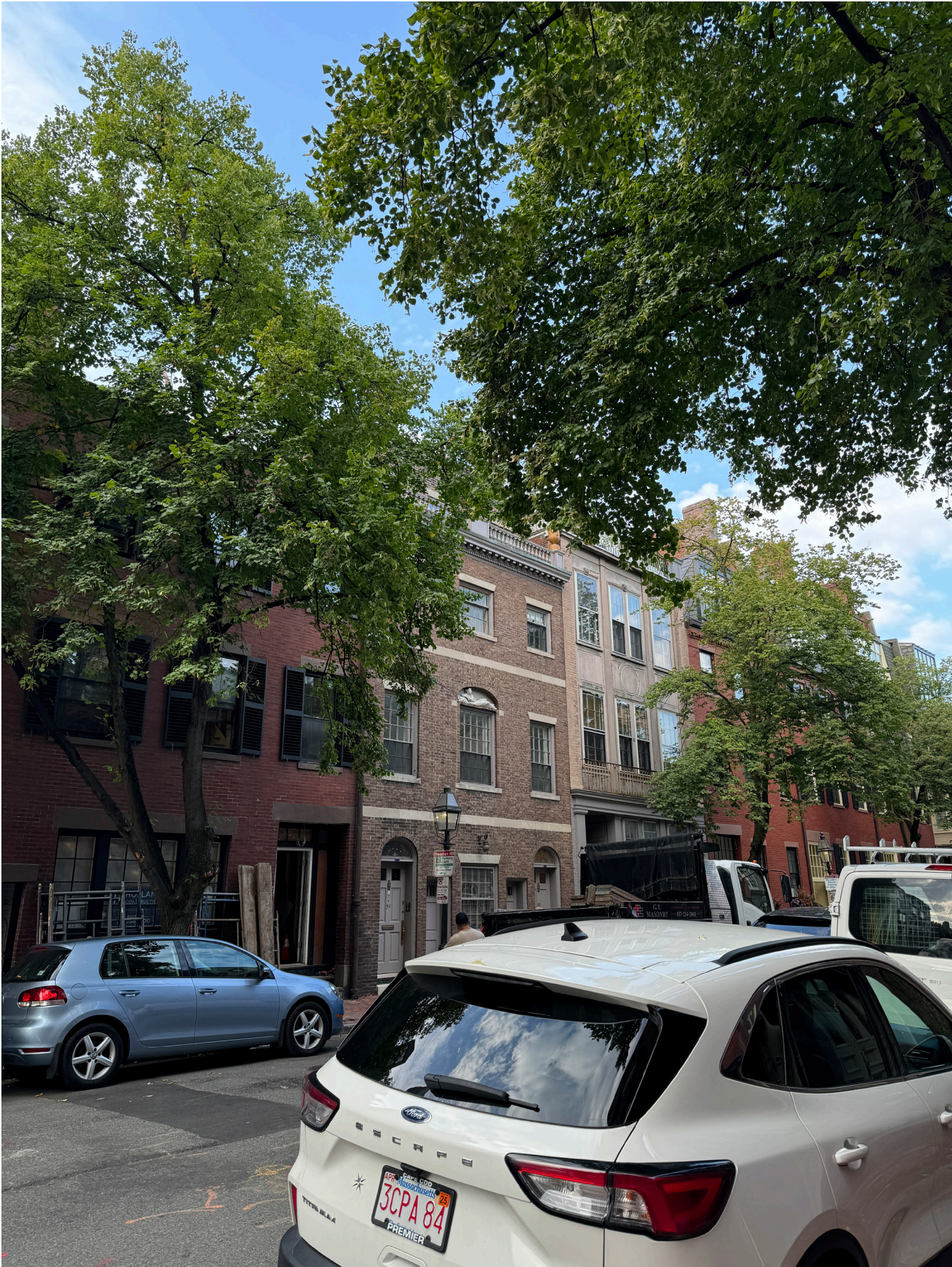
CHESTNUT ST VIEW OF FACADE FROM EAST
