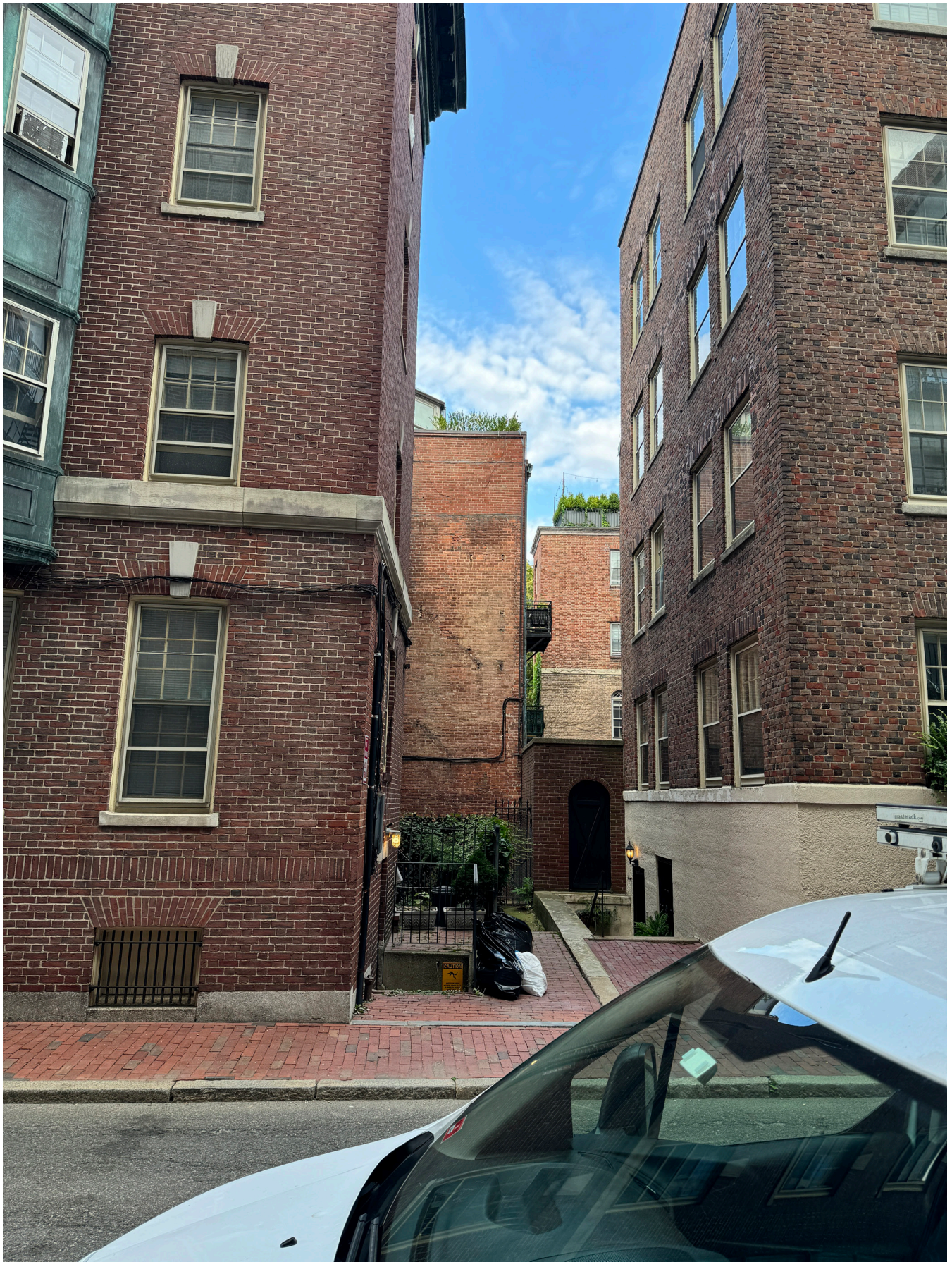
RIVER ST VIEW OF REAR ELL
