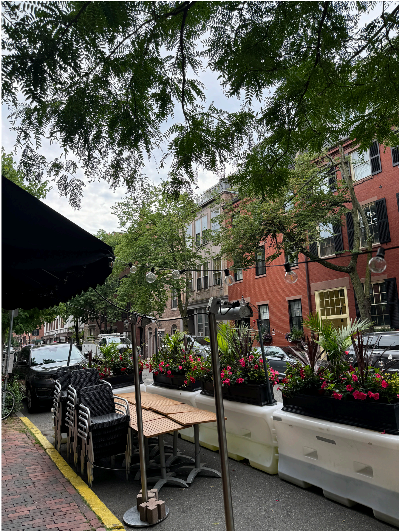
CHESTNUT ST VIEW OF FACADE FROM WEST
