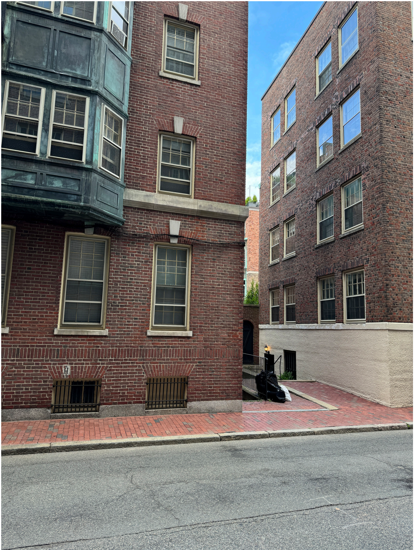
RIVER ST VIEW OF REAR PORTION OF PARTY WALL
