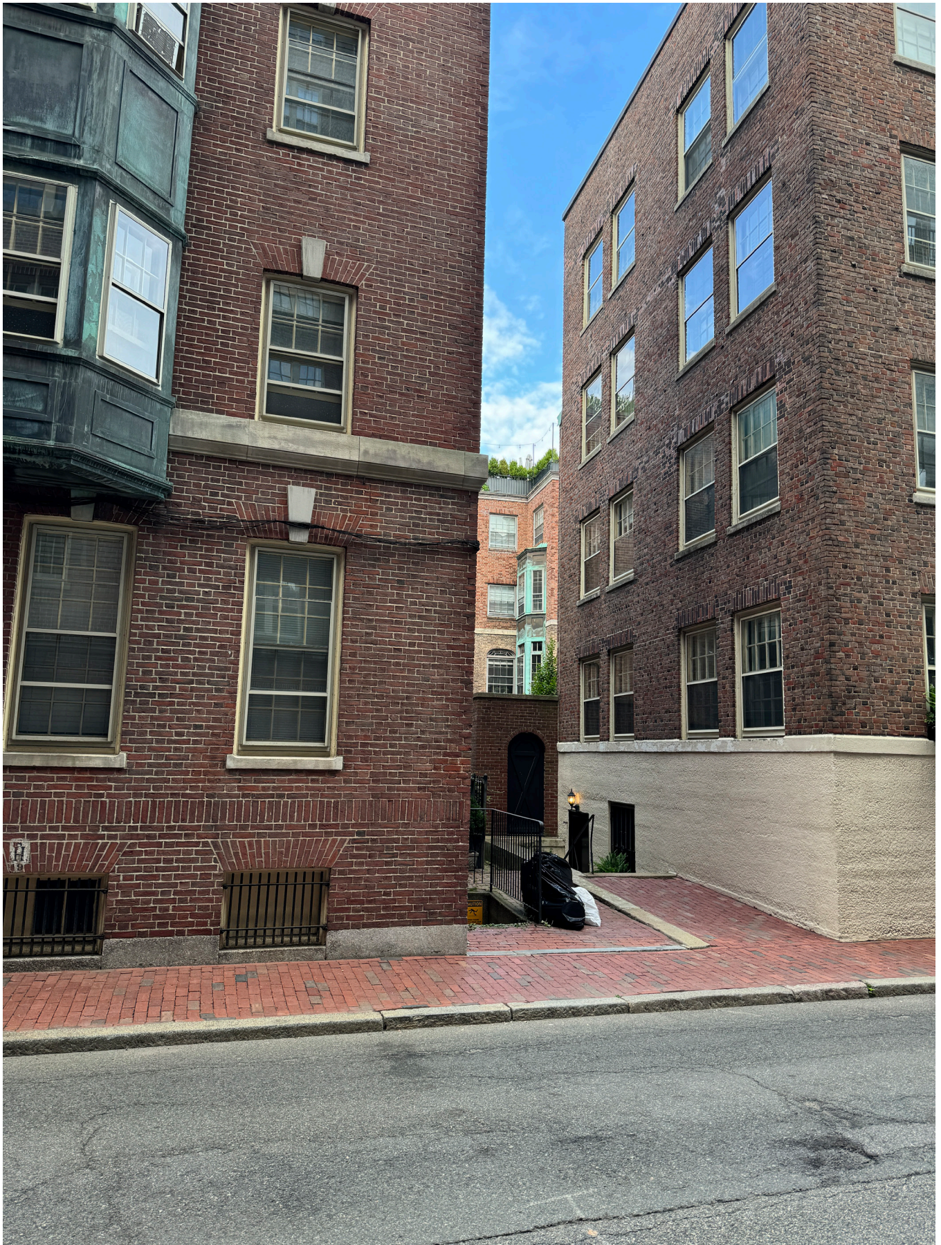
RIVER ST VIEW OF REAR ELL/ REAR WALL
