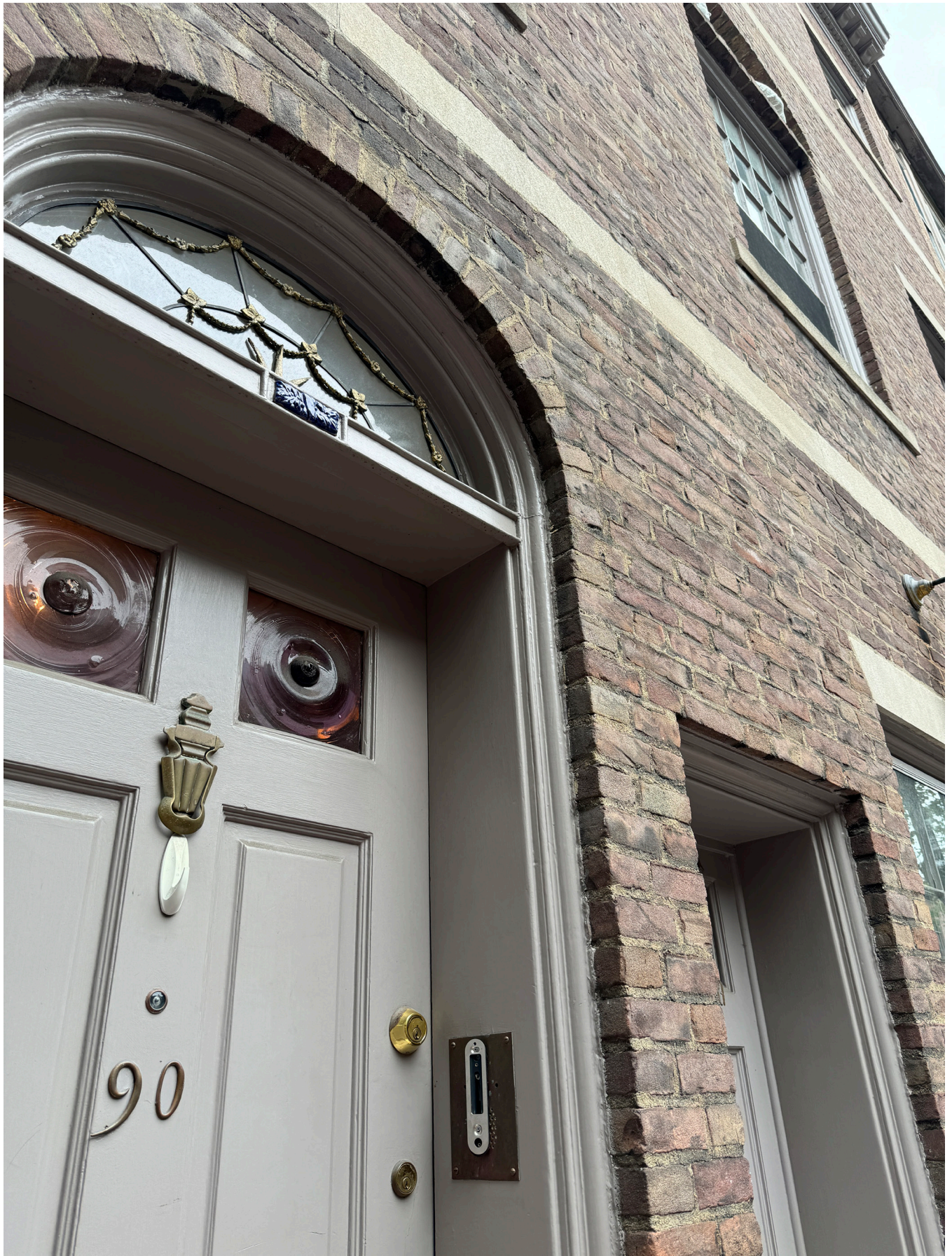
EAST FRONT DOOR CLOSE UP
