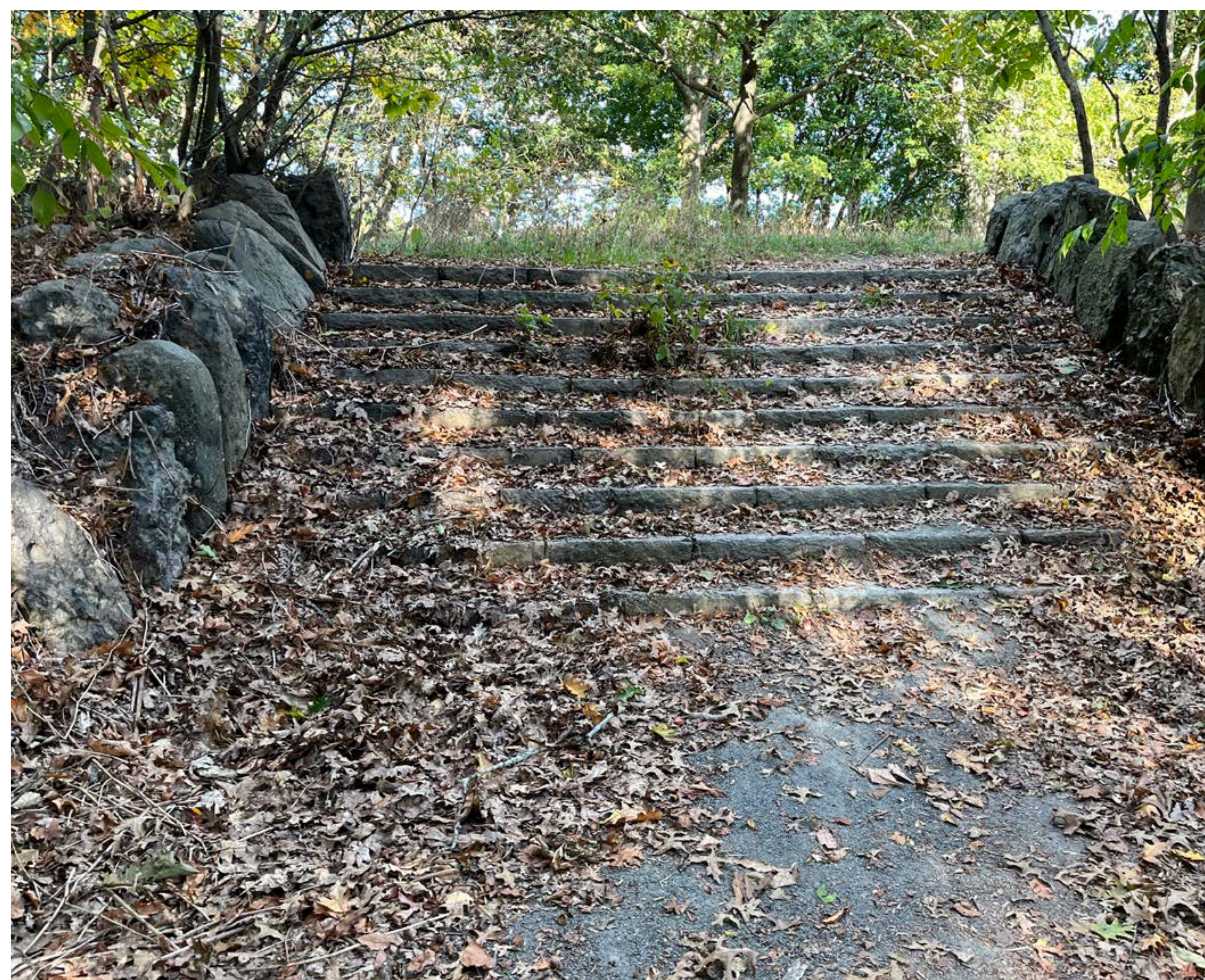
Disconnected entries, steep slopes, and stairs limit the accessibility of the Overlook.
