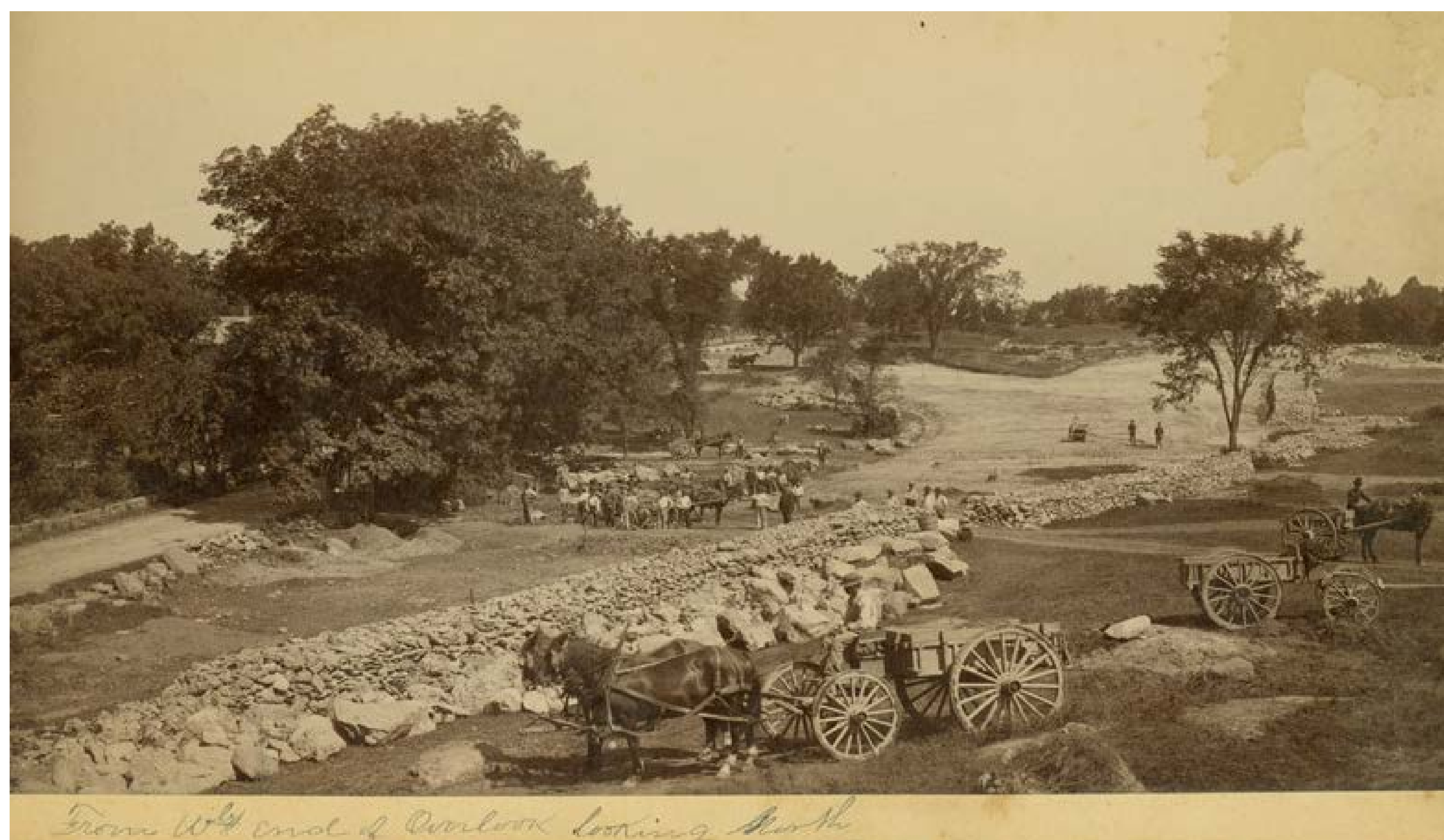
1 1887 construction of the Overlook.
