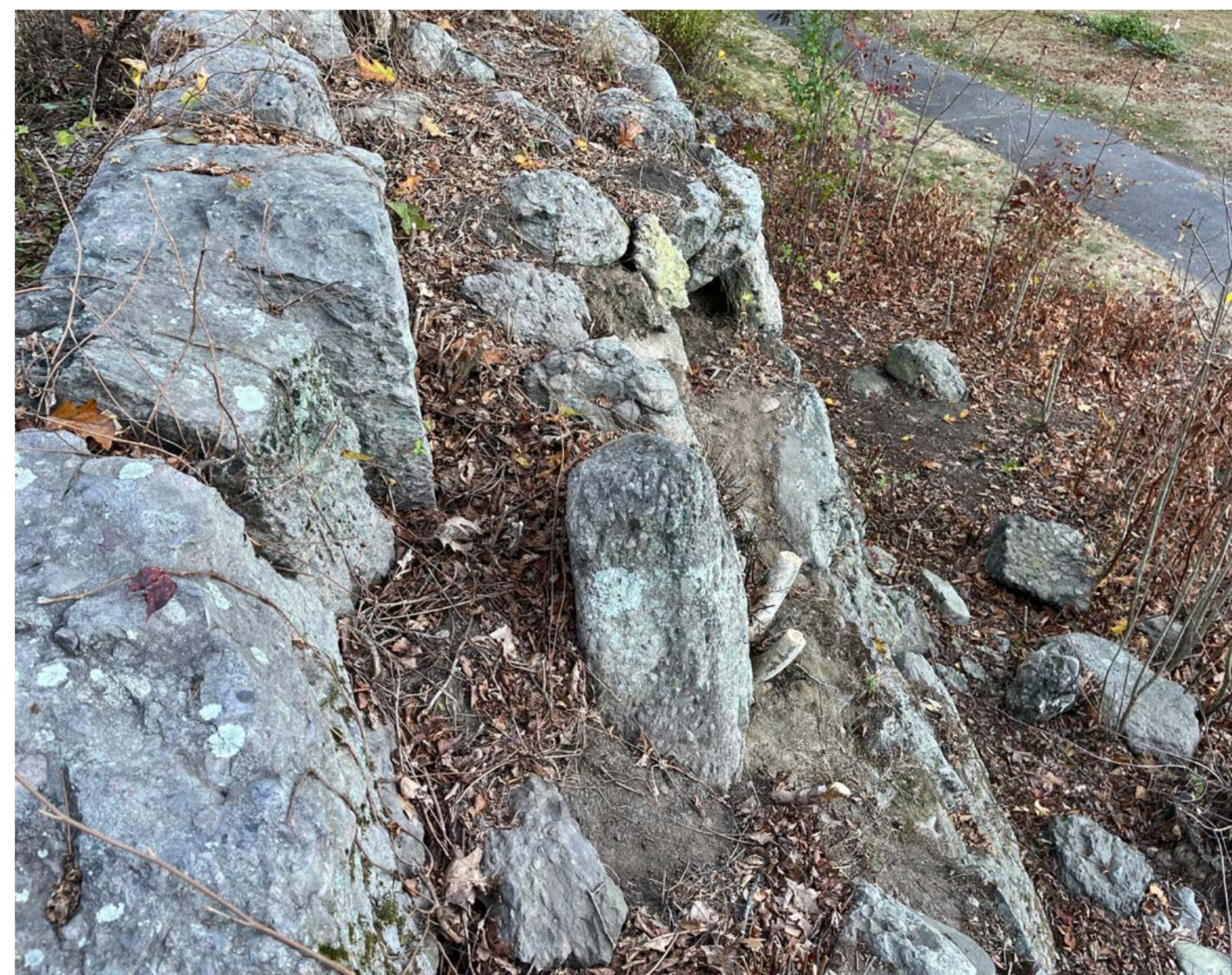
The puddingstone walls and ruins define the Overlook. The walls and ruins are in need of stabilization in some areas as many stones have become loose or dislodged.
