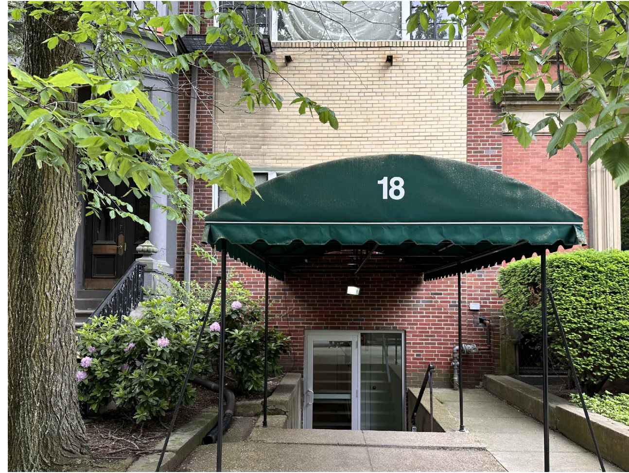
EXISTING FRONT ENTRANCE & GARDEN
