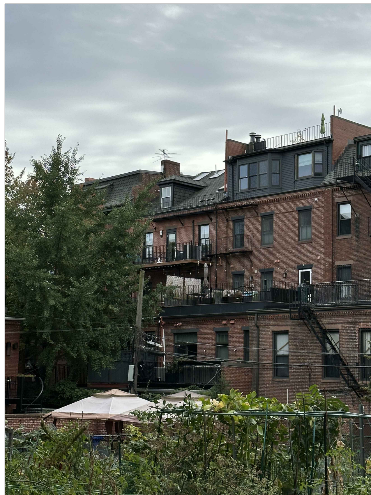
EXISTING SIMILAR DECKS ON NEAR BY ABUTTERS IN ALLEY
