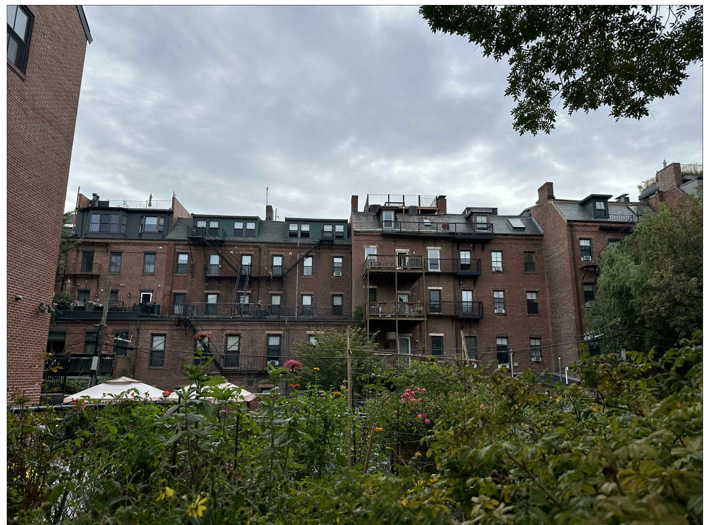
EXISTING SIMILAR DECKS ON NEAR BY ABUTTERS IN ALLEY
