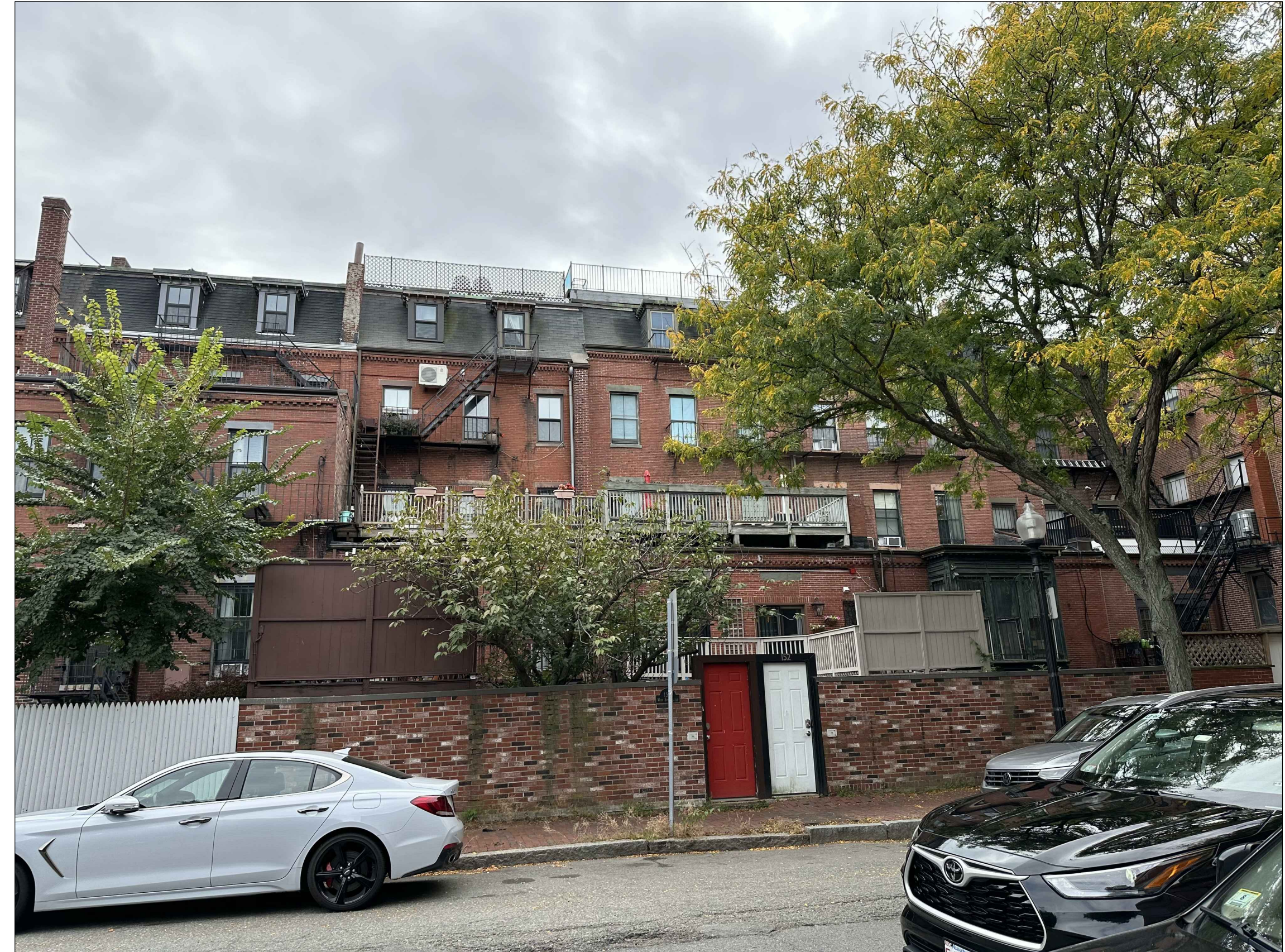
EXISTING REAR WALL/ PROPOSED DECK LOCATION
