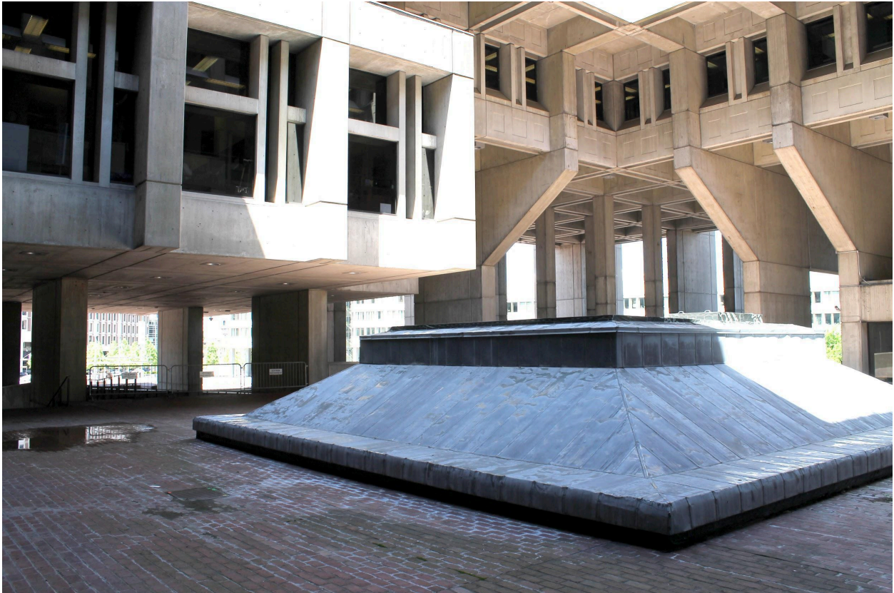
Figure 13. Pyramidal skylight in the central courtyard. (2018)
