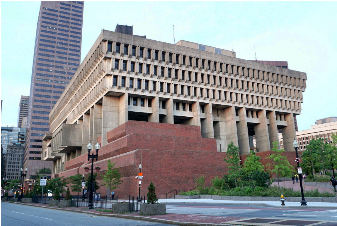
Figure 6. Brick terracing at the northeast corner of the building, June 2023. Photo credit: Building Conservation Associates.
