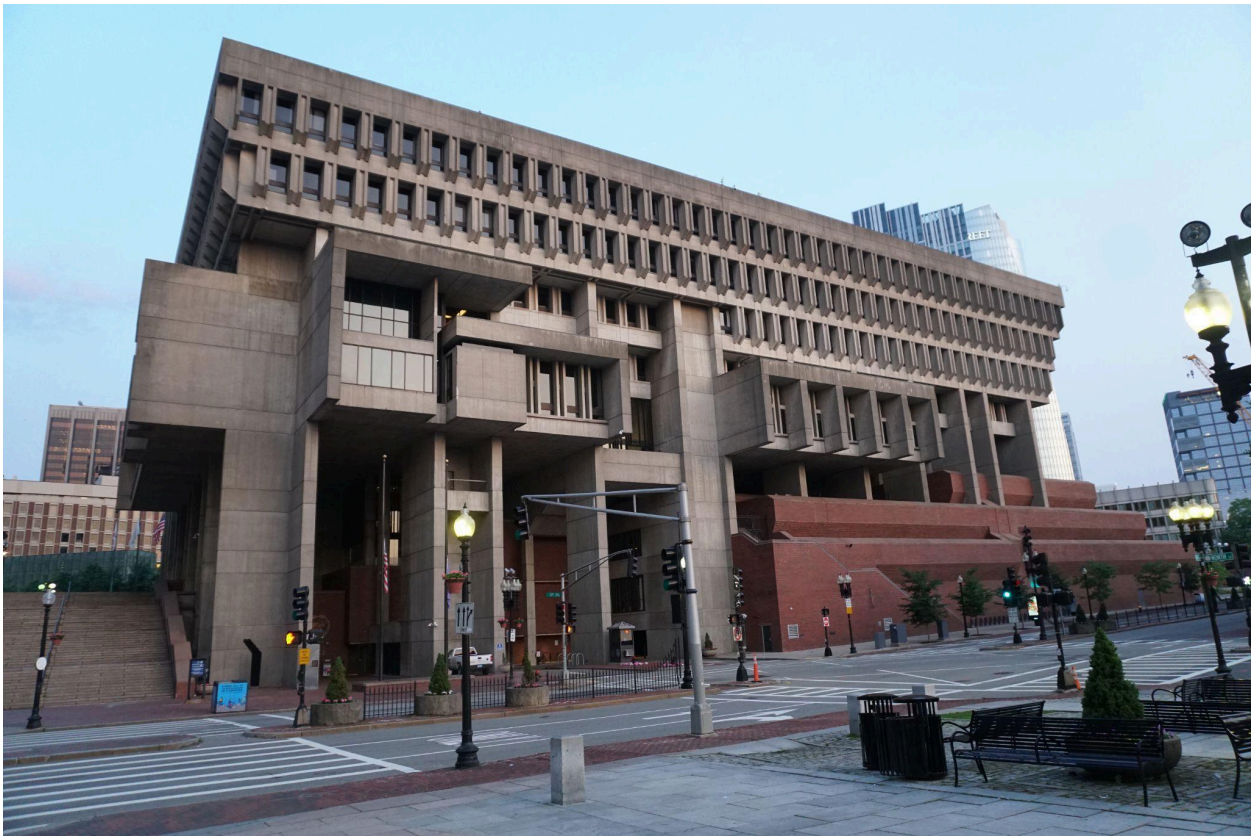
Figure 4. East elevation, June 2023. Photo credit: Building Conservation Associates.
