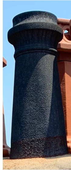
EXISTING CHIMNEY POT TYPE 1
