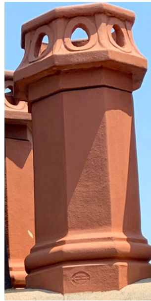
EXISTING CHIMNEY POT TYPE 2
