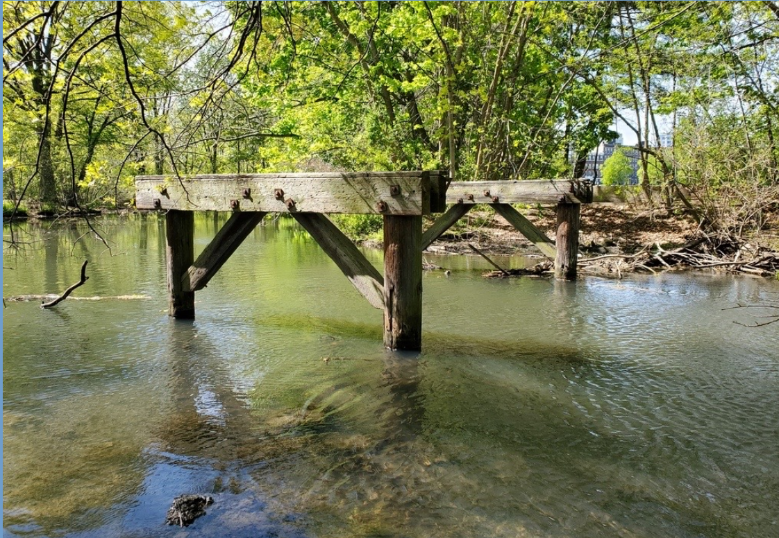
Bridge Prior to Complete Demolition
