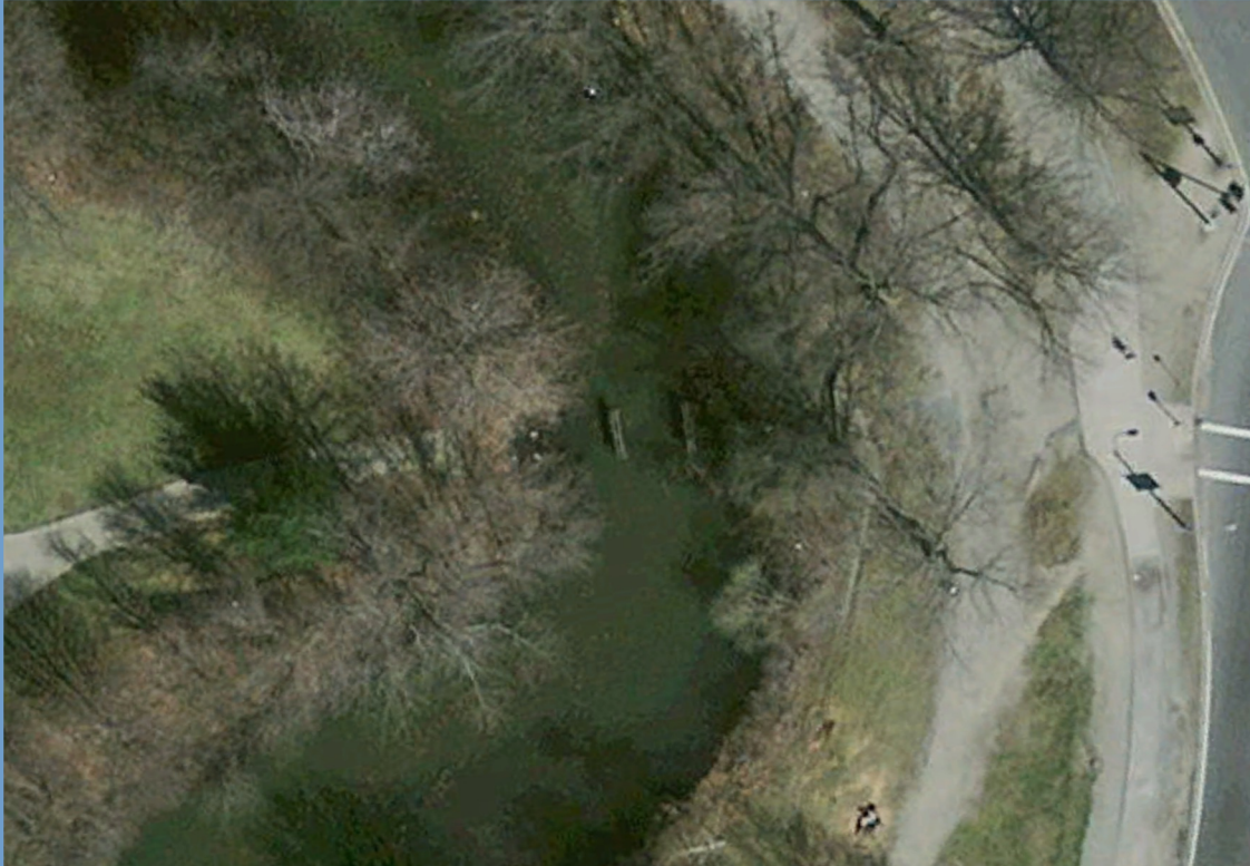
Bridge Prior to Complete Demolition
