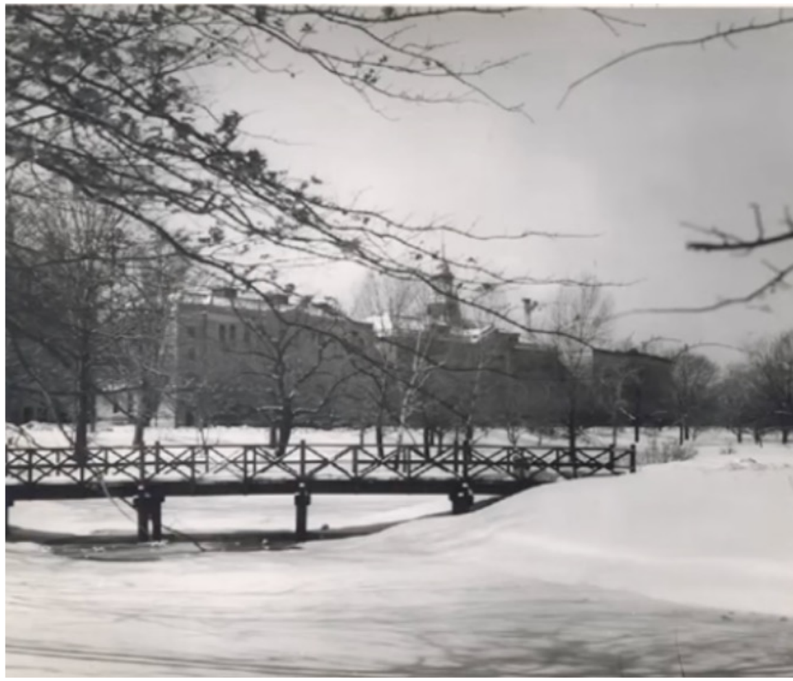
Evans Way Bridge, 1950's
