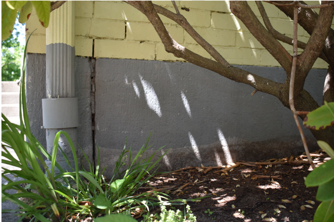
Figure 7. Daniel Withington House, hammered granite foundation detail, looking northwest (The Public Archaeology Laboratory, Inc. 2021).
