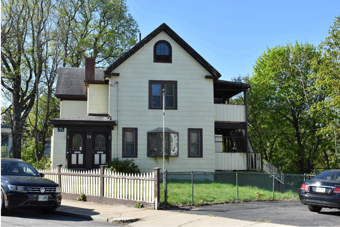
Figure 4. Daniel Withington House, north elevation, looking south from Ashland Street (The Public Archaeology Laboratory, Inc. 2021).
