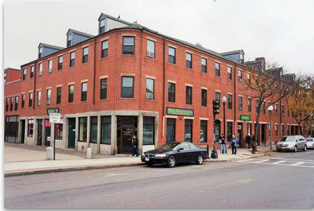
Woodbury مبنى East Boston
