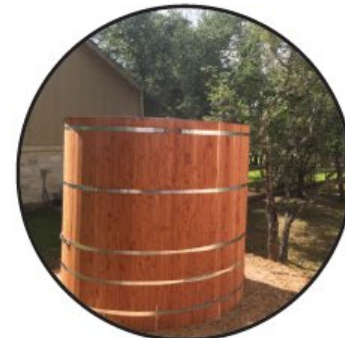
Rainwater harvesting 3000+ gallon capacity
