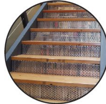
Metal risers thermally modified oak treads stained brown
