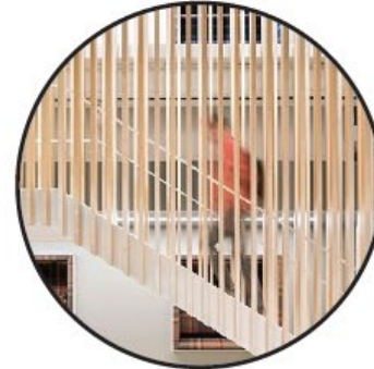
Thermally modified stair enclosure stained brown
