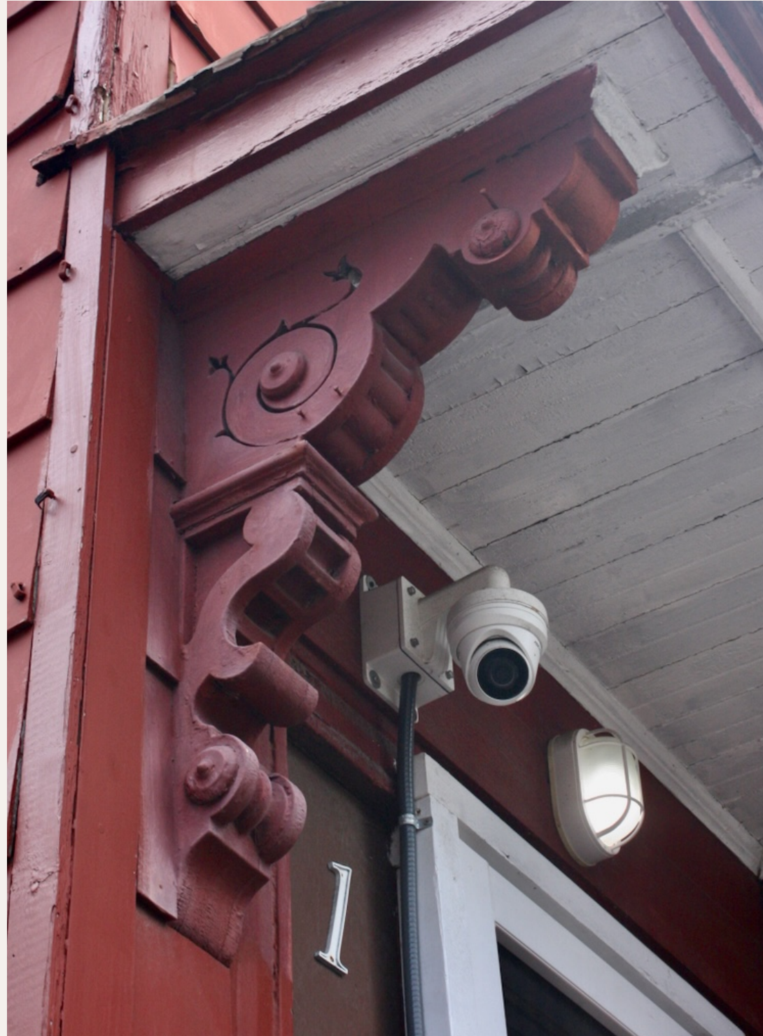
Photo: West entrance: Bracket detail
