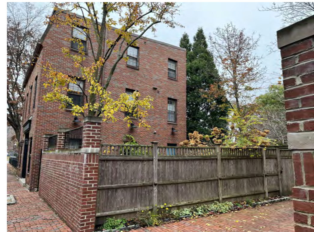
PARKING AREA FACADE (HISTORIC WILKES STREET)
