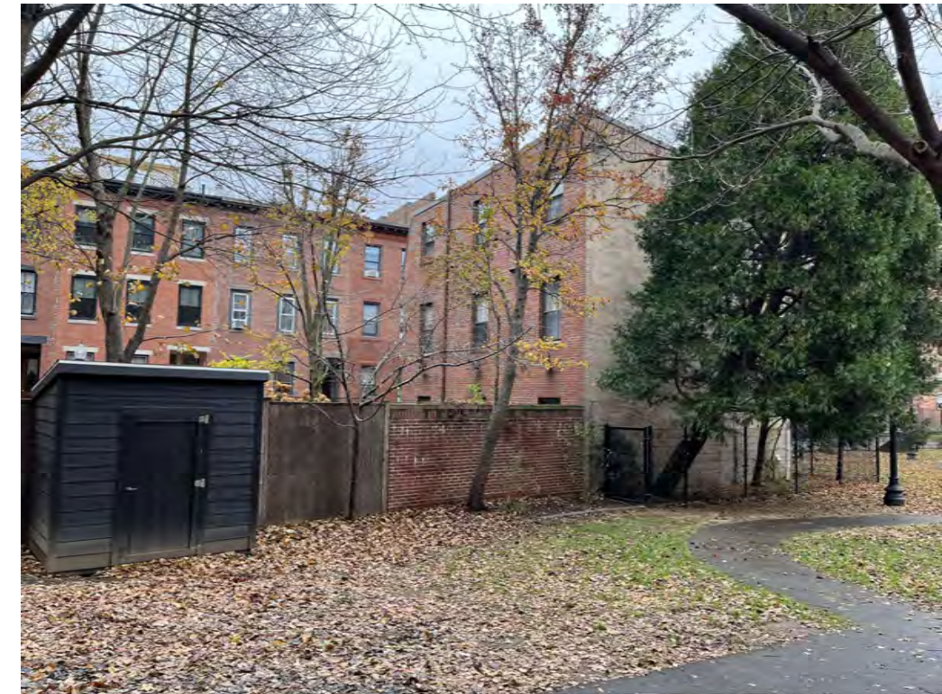
PETERS PARK FACADE
