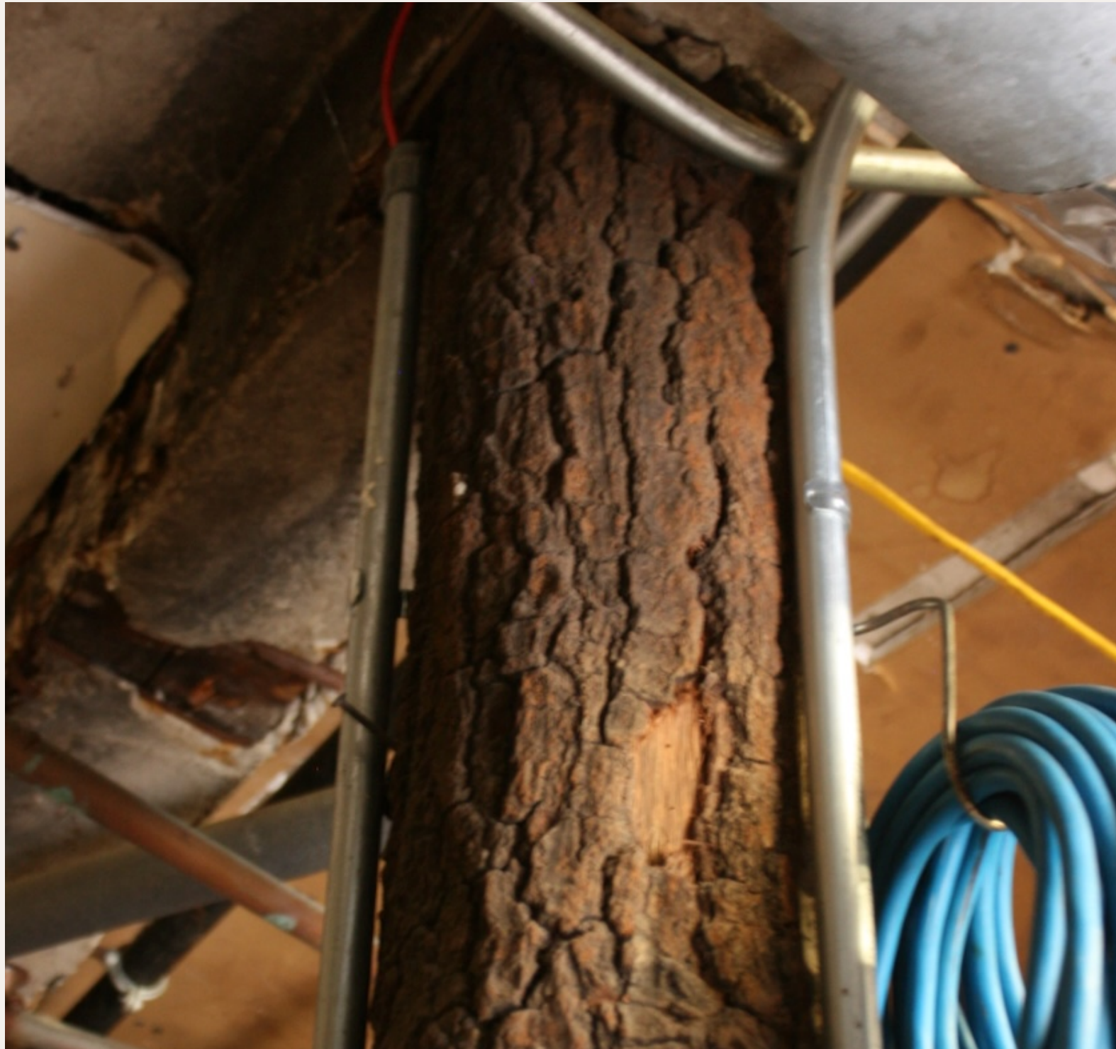
Photo: Tree trunk post in basement
