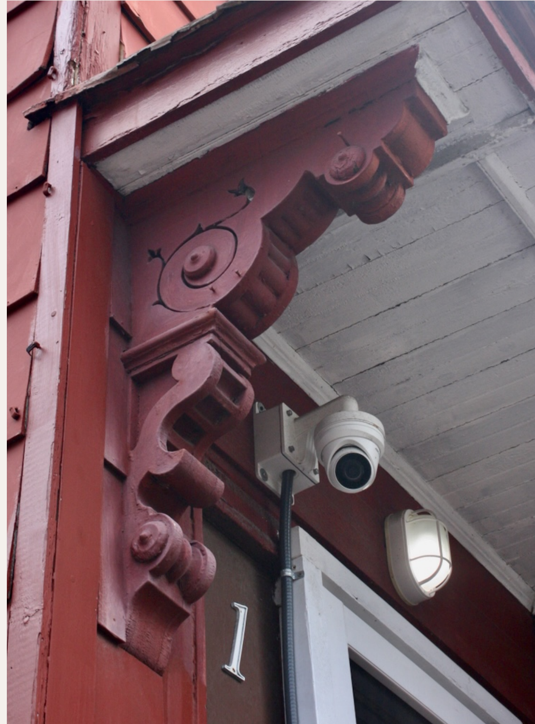
Photo: West entrance: Bracket detail
