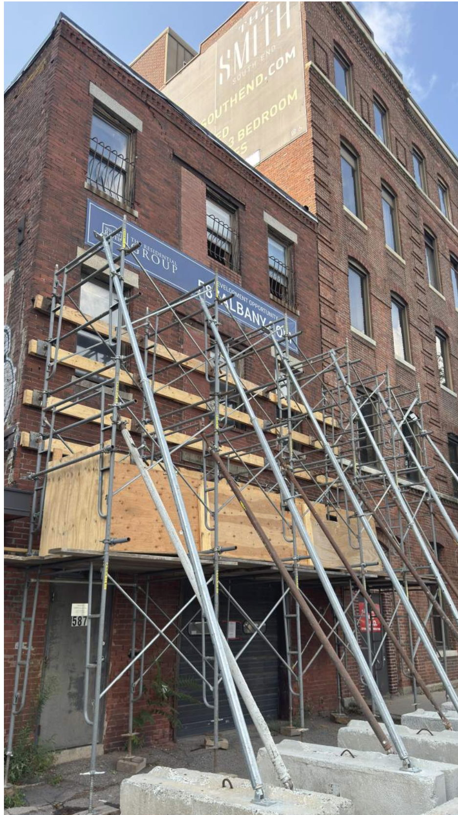
FACADE BRACING IN PLACE
