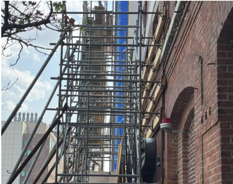
BRACING IN PLACE AGAINST BOWED MASONRY WALL
