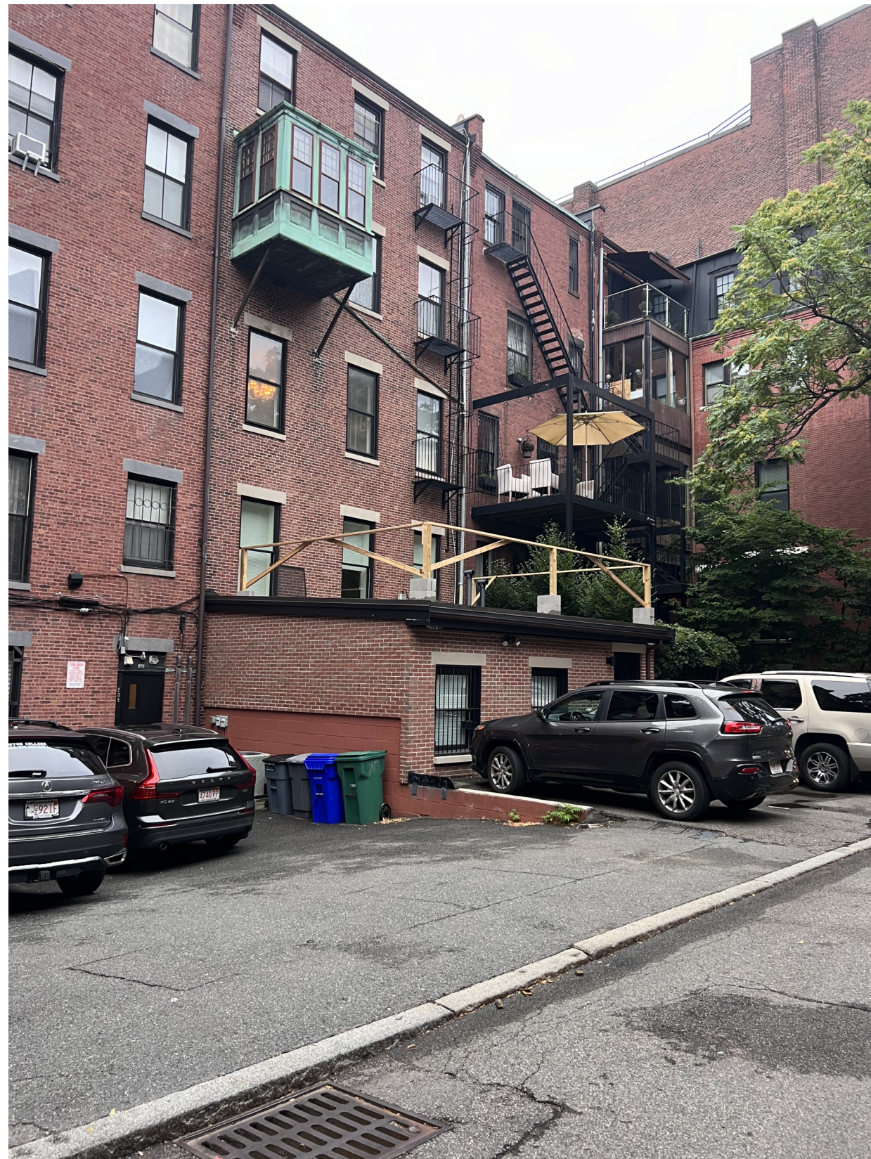
West Elevation Mockup
