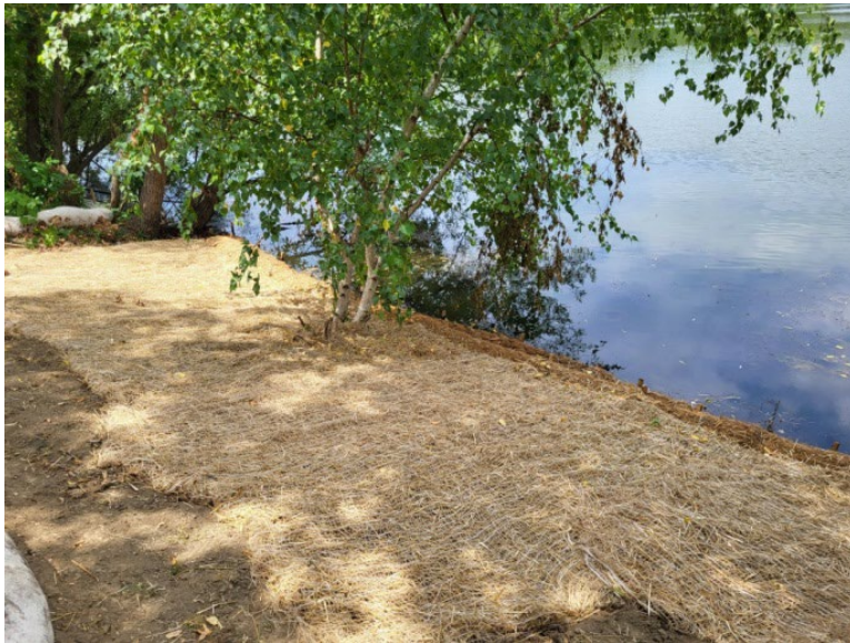
Erosion control matting being installed
