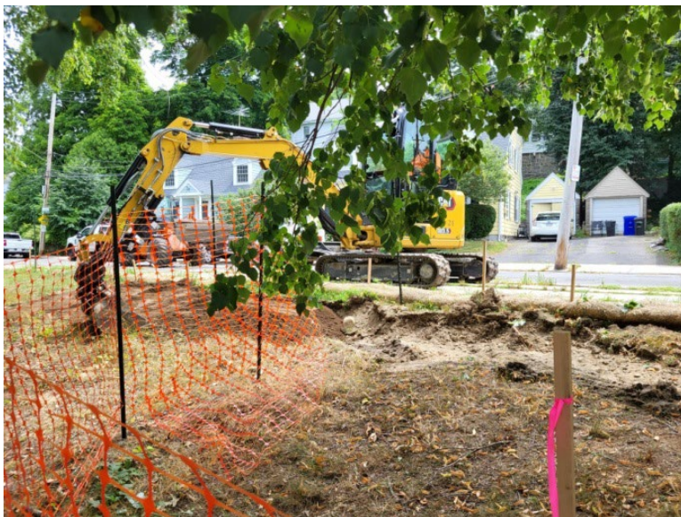
Preparing the existing soil to receive new topsoil and turf seed
