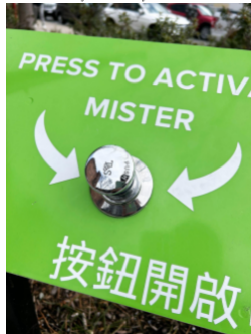
Example of a metered water valve. This type of valve is set to dispense water for a defined amount of time, meaning there is no risk of water being left on.
