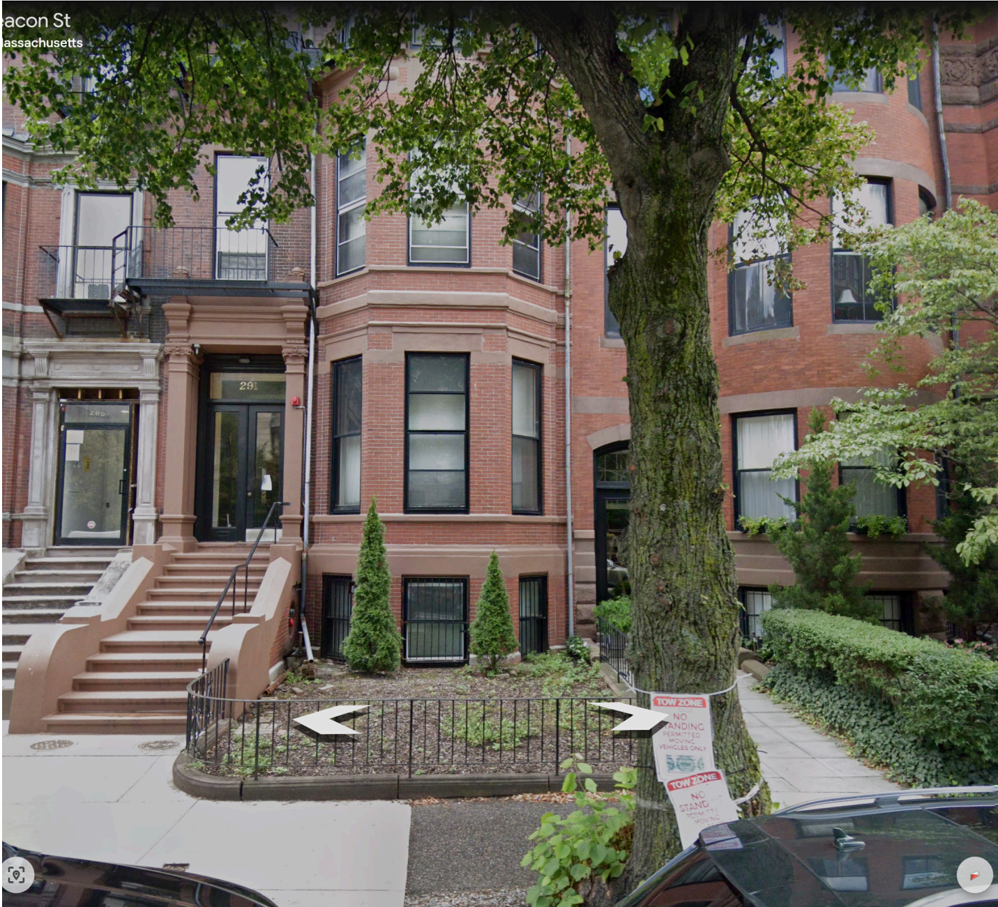
STREET VIEW OF EXISTING FRONT FACADE @ 291 BEACON ST
