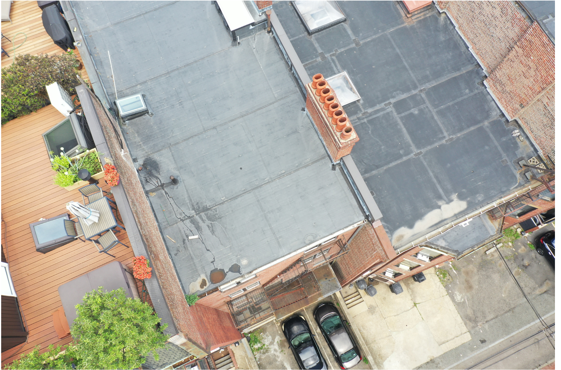
EXISTING ROOF @ SOUTH SIDE @ 291 BEACON ST
