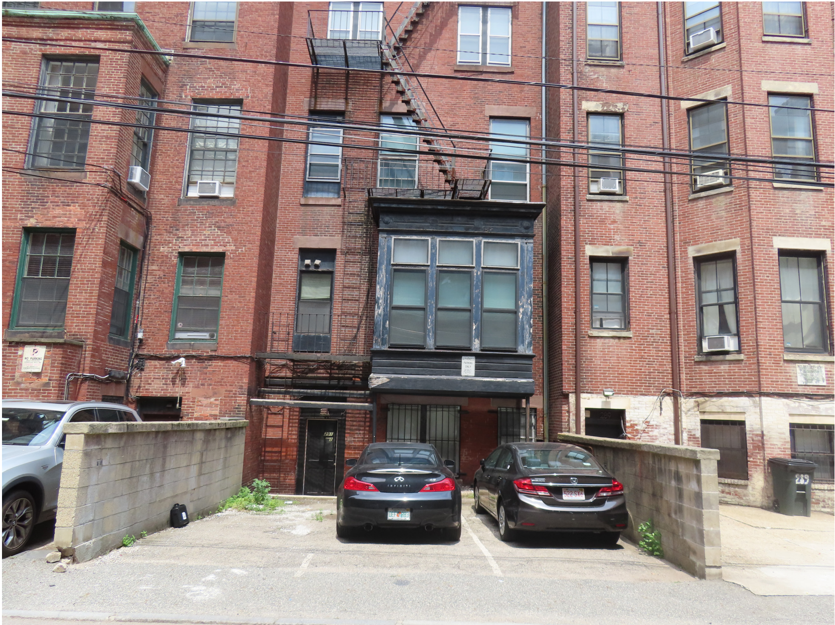
EXISTING LOWER SECTION OF REAR FACADE@ 291 BEACON ST
