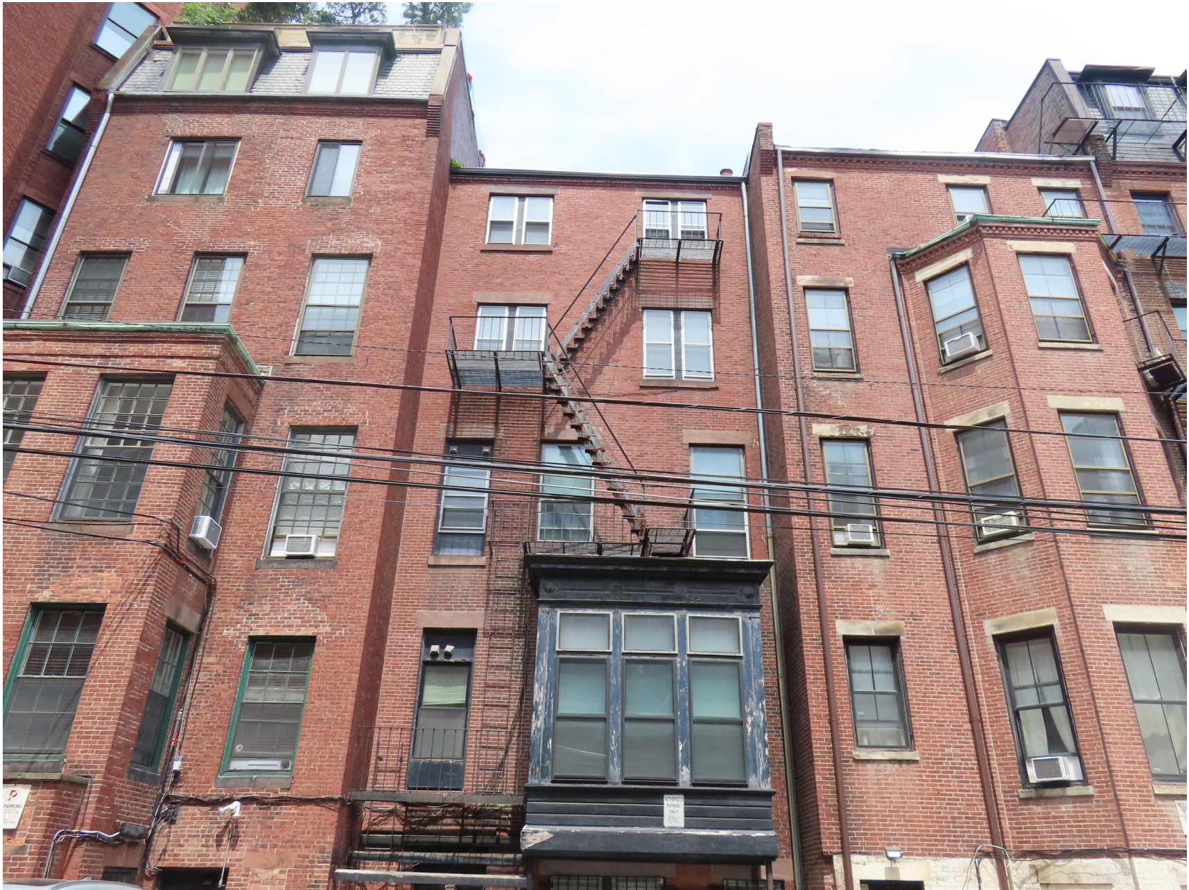
EXISTING UPPER SECTION OF REAR FACADE@ 291 BEACON ST
