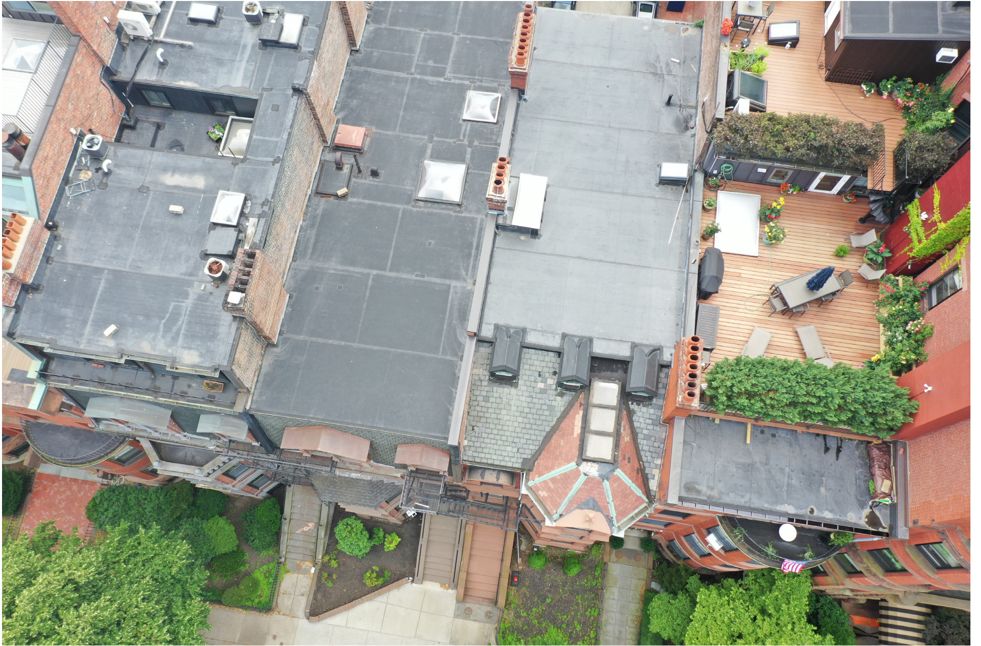
EXISTING ROOF @ NORTH SIDE @ 291 BEACON ST
