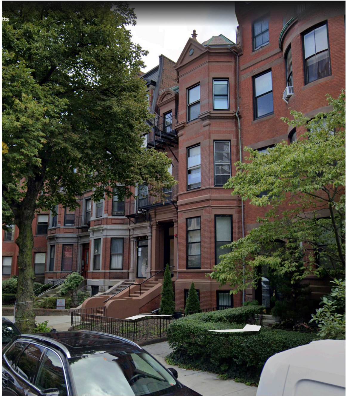
NORTH WEST VIEW OF EXISTING FRONT FACADE @ 291 BEACON ST
