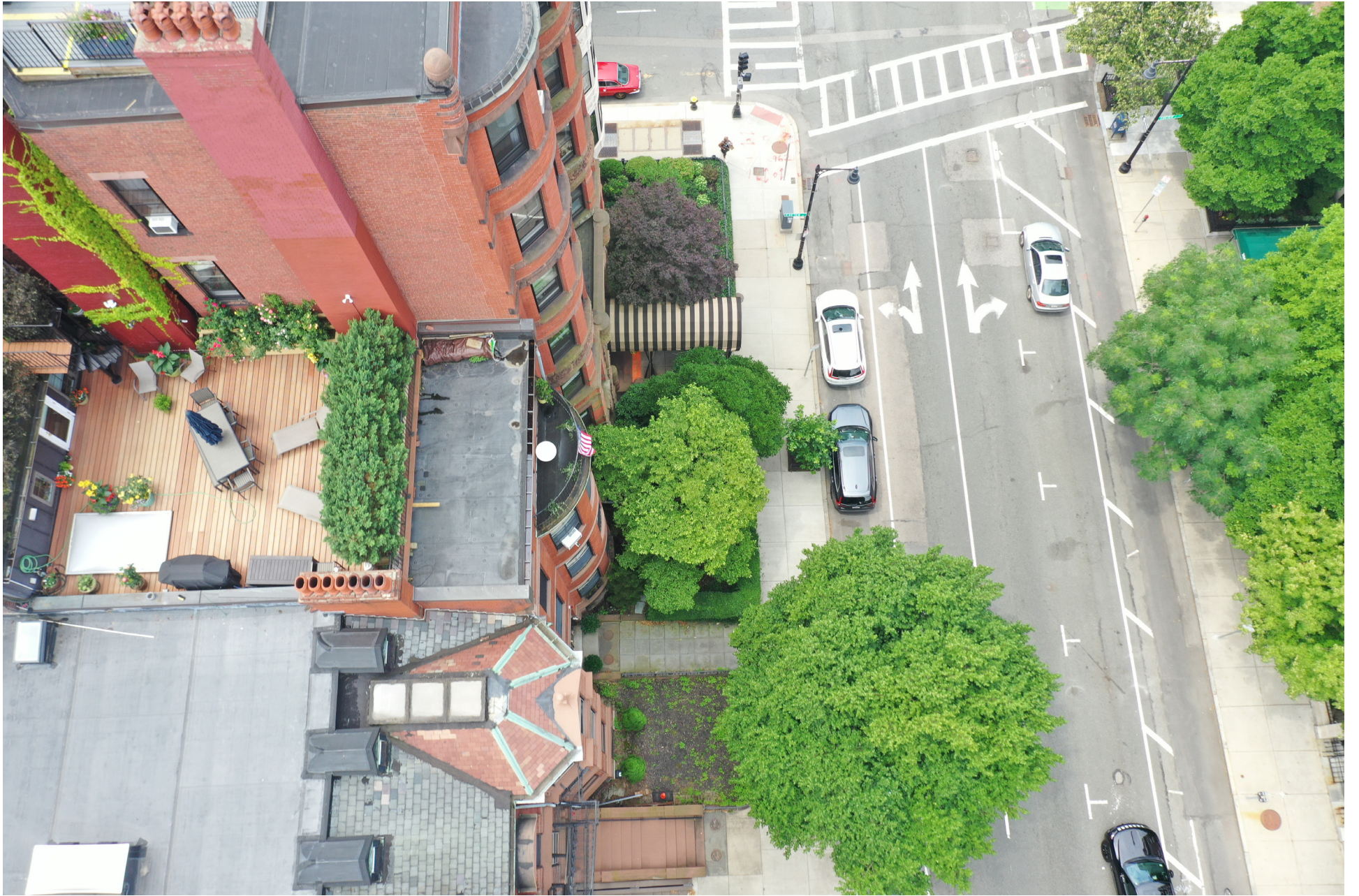
EXISTING ROOF @ NORTH SIDE @ 291 BEACON ST
