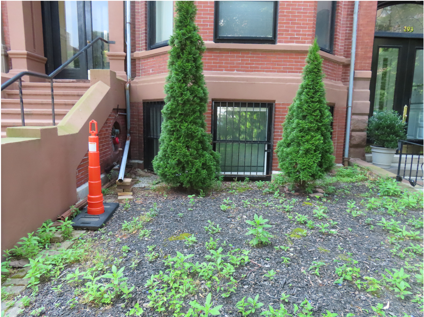
EXISTING FRONT FACADE CLOSE UP@ 291 BEACON ST
