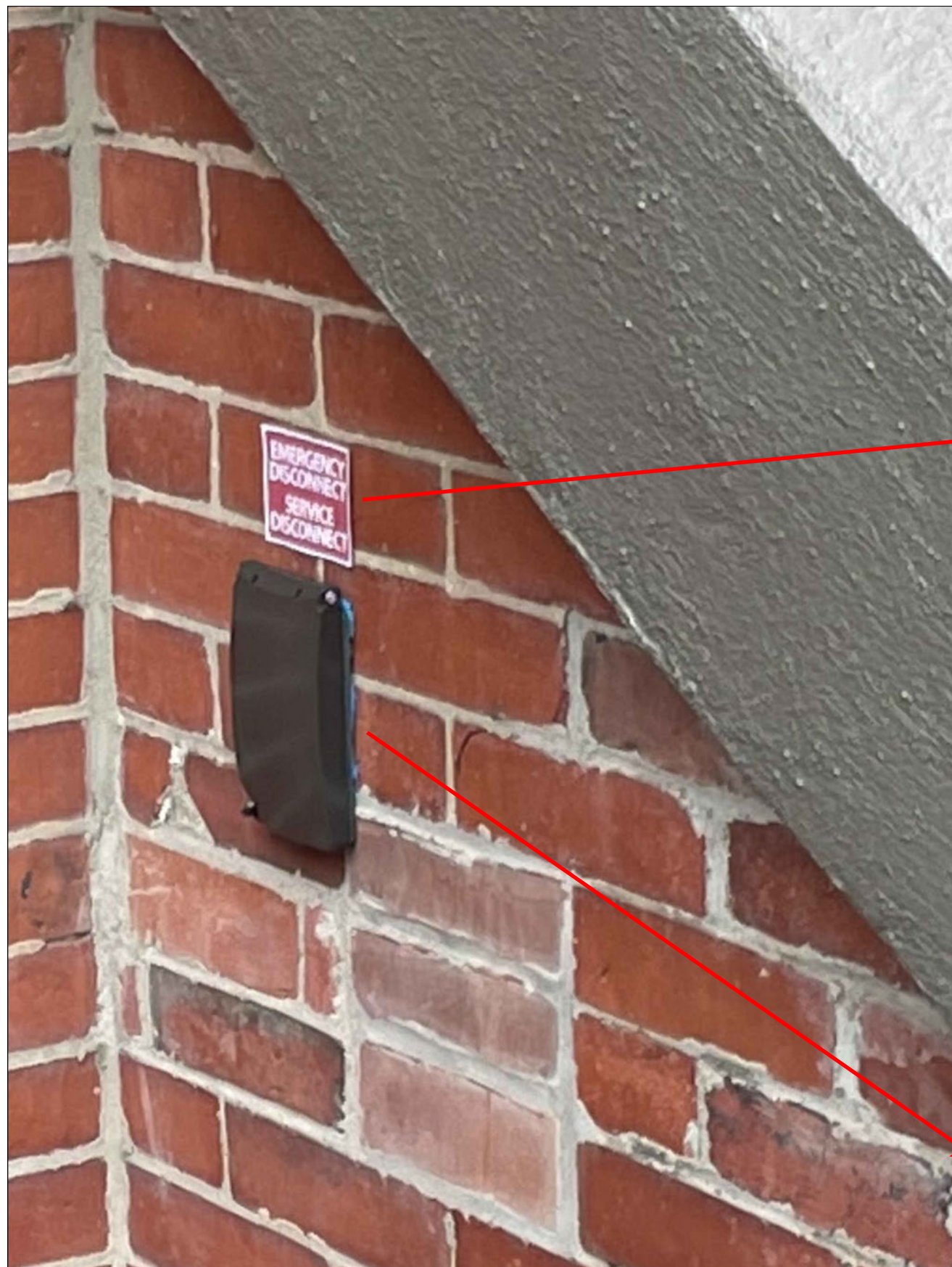
1 PROPOSED EMERGENCY ELECTRICAL SHUTOFF DETAIL
