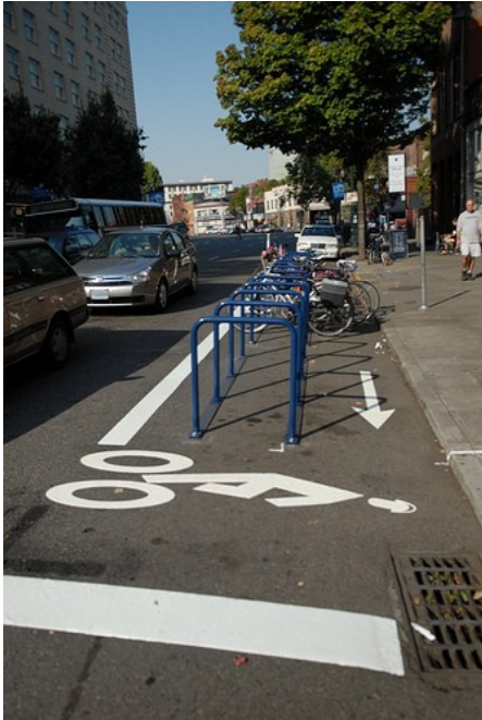
Example of bike corral installation. Corrals typically can park 10 to 20 bicycles, using space otherwise occupied by one or two cars.
