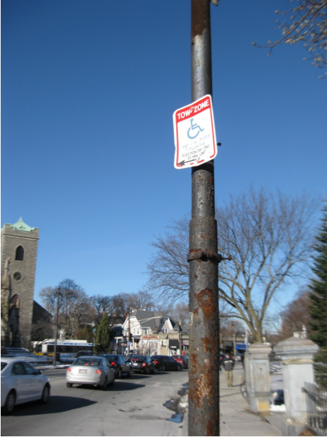
The City of Boston has formally requested that the MBTA remove the remaining catenary poles.
