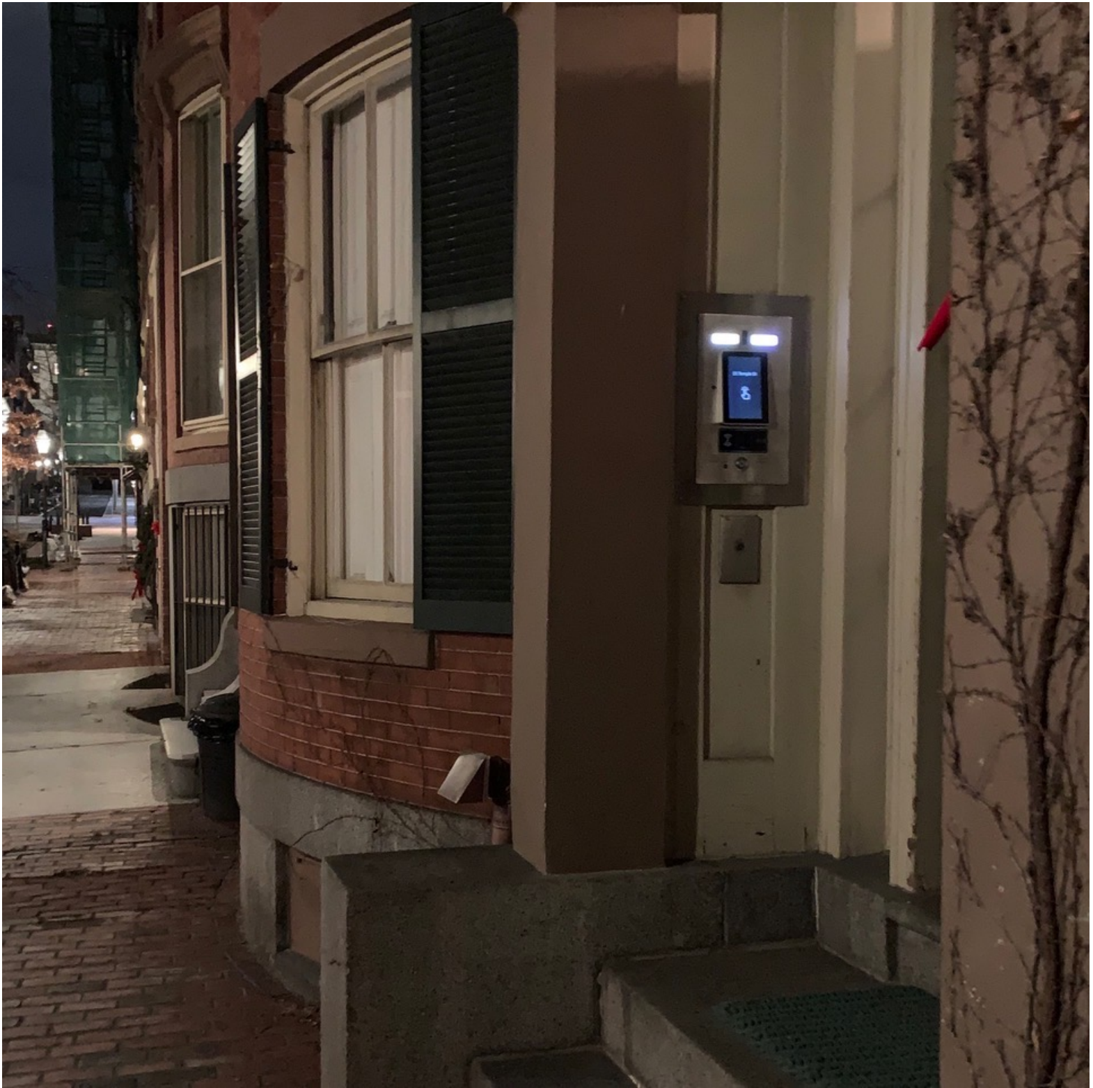
Existing Butterfly Intercom to Left of Door
