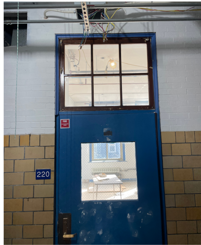
UNCOVERED CLERESTORY WINDOWS
