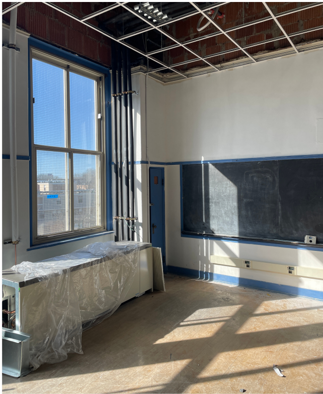
NEW CEILING PROGRESS
