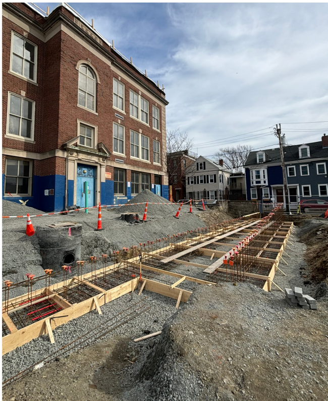
ONGOING SITE WORK
