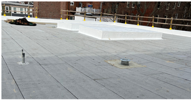
NEW ROOF INSTALLED
