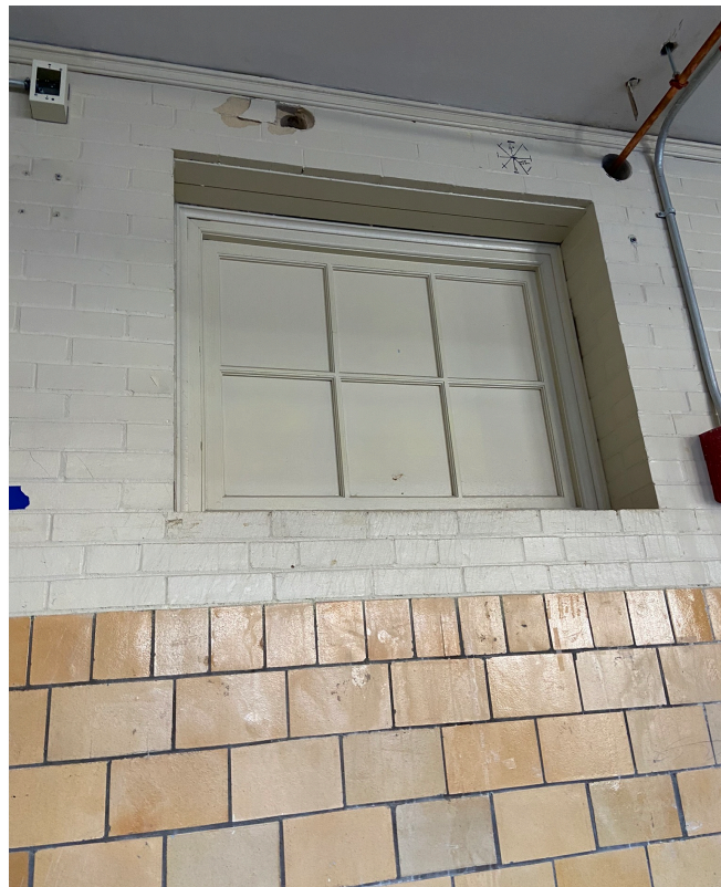
EXISTING CLERESTORY WINDOWS
