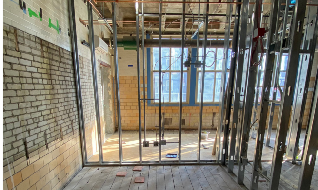
NEW WALLS UNDER CONSTRUCTION
