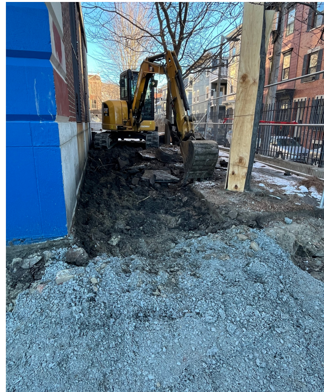
ONGOING LANDSCAPE WORK
