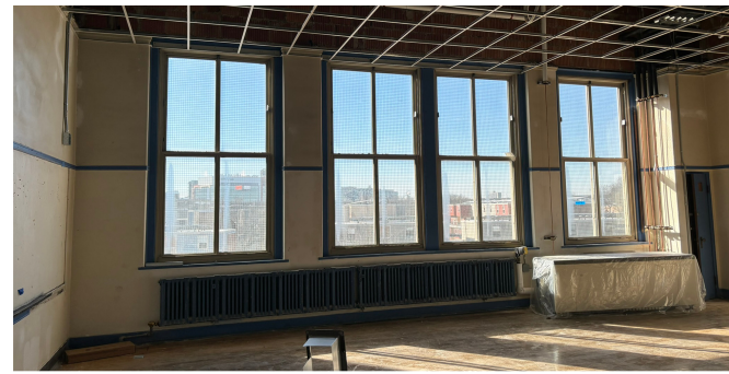
NEW CEILING PROGRESS
