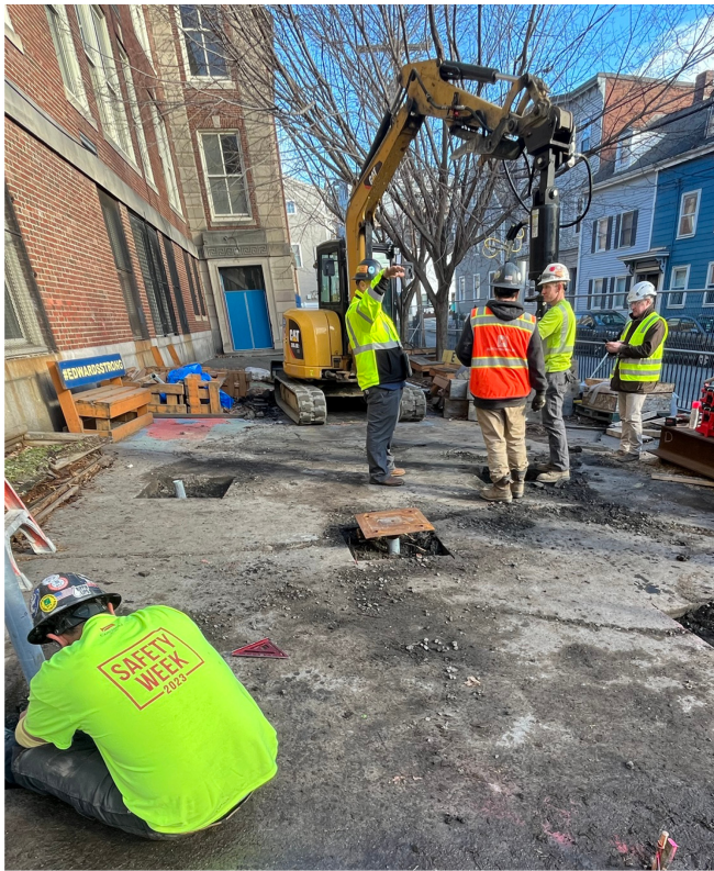
ONGOING LANDSCAPE WORK
