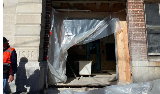
NEW ENTRANCE FOR ELEVATOR ACCESS
