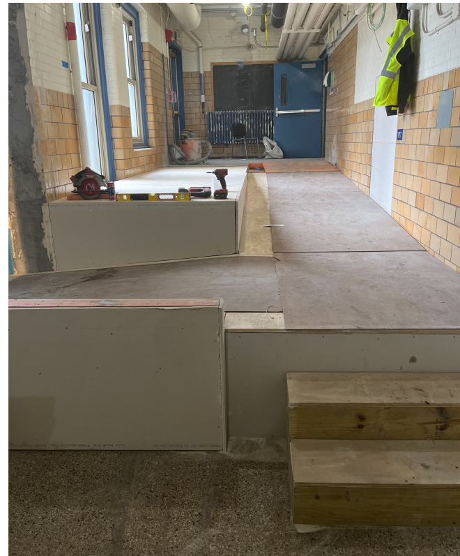
NEW RAMP PROGRESS
