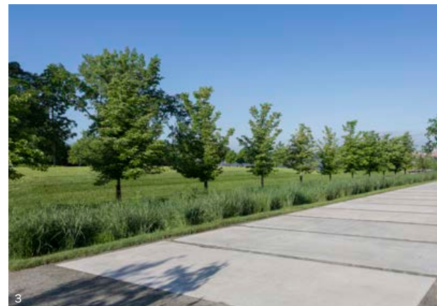
3 Vegetated swale at the edge of parking.
