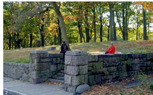
2 Medium Entrance: Historic stone masonry at the old Refectory.
