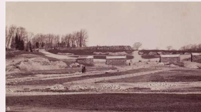
Field stones uncovered during park construction were salvaged for the perimeter wall.
