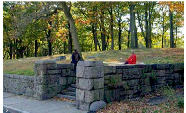
2 The existing entrance on Blue Hill Ave between McLean and Charlotte Streets.
