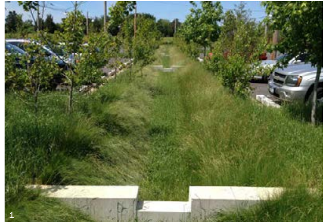
1 Vegetated swale in the center of parking.
