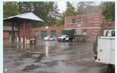
Today the maintenance yard is a complex of buildings, stables, and greenhouses, and serves Boston's entire park system
