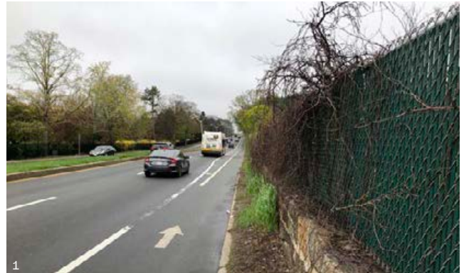
The low historic puddingstone perimeter wall with a chain link fence and no sidewalk along Morton Street, a state highway.
