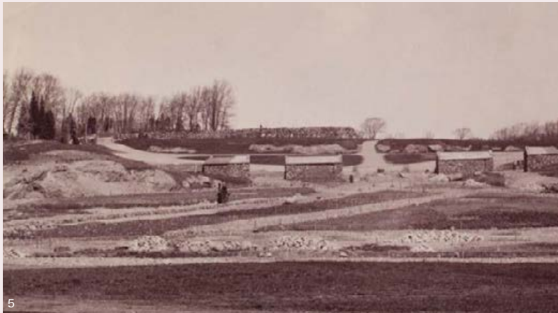
5 Field stones uncovered during park construction were salvaged for the perimeter wall.
