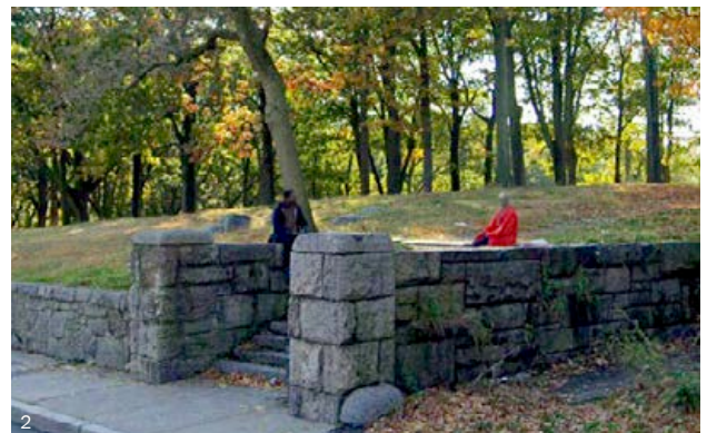
Medium Entrance: Historic stone masonry at the old Refectory.
