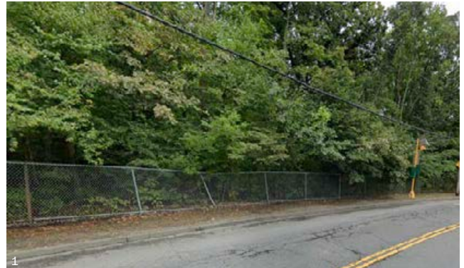
Chain link fence along Williams Street.
