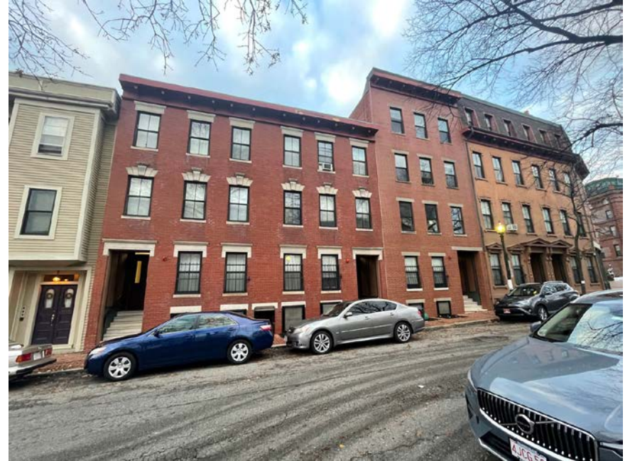
On Dudley St Across From Site
