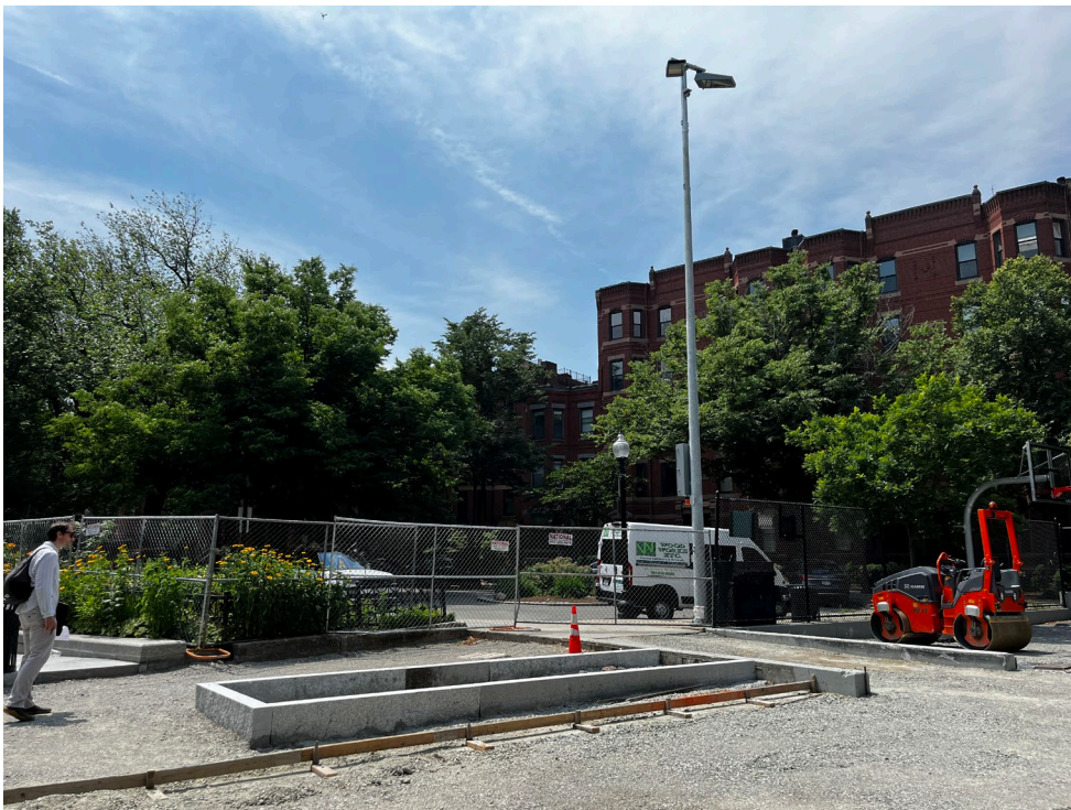
Granite curbing has been installed
