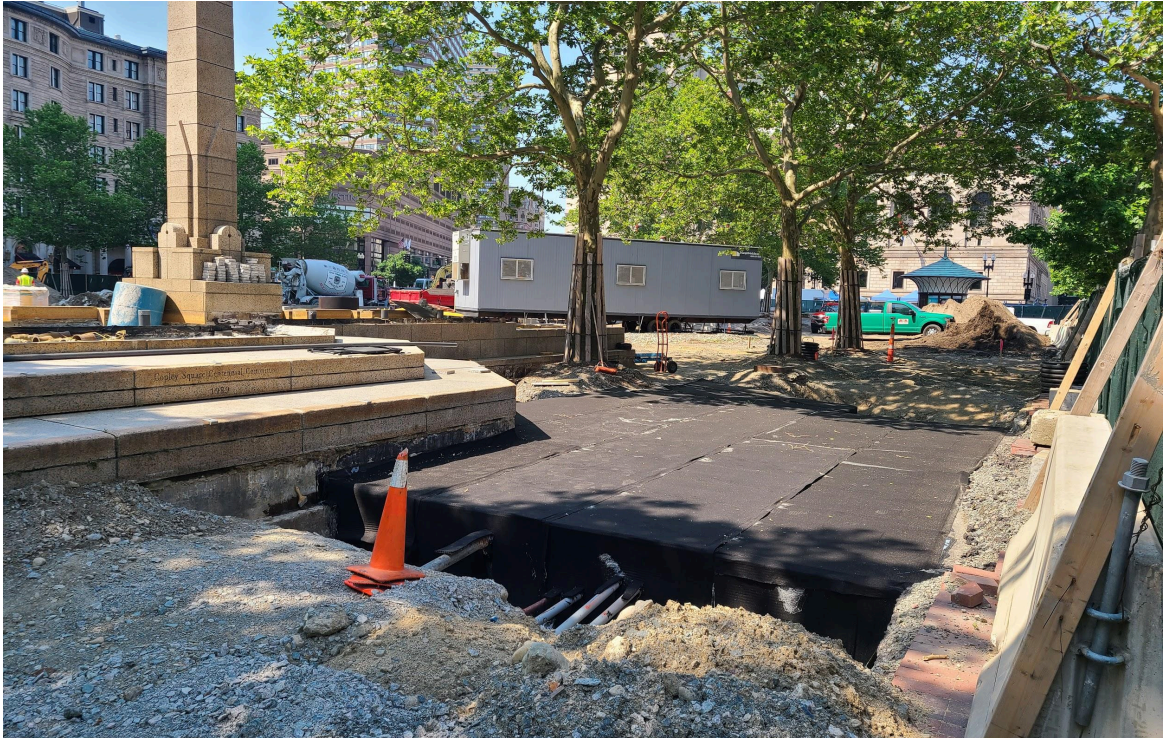
Waterproofing the roof of the fountain vault.
