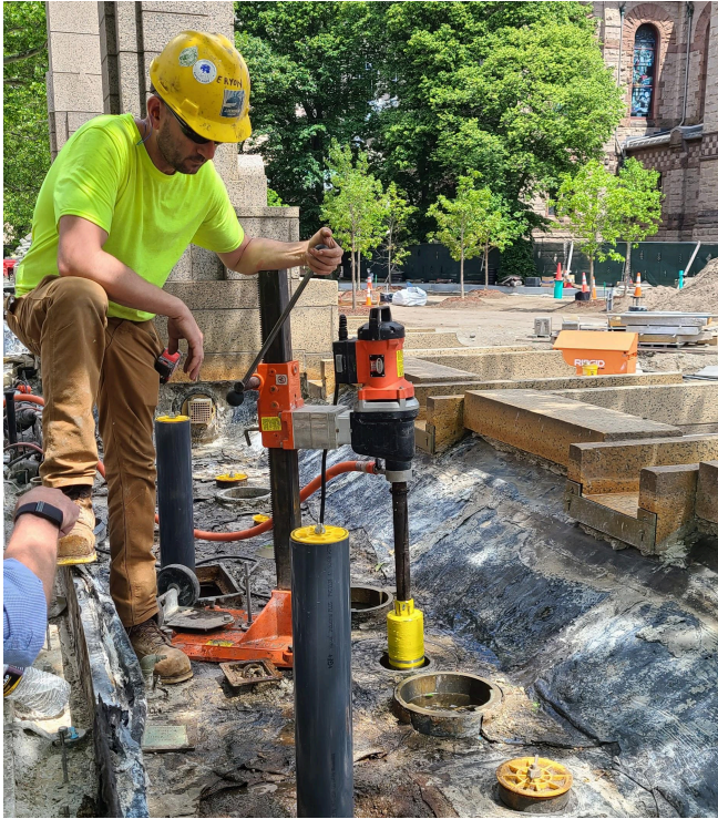
Replacing the piping to the nozzles in the upper fountain pools.
