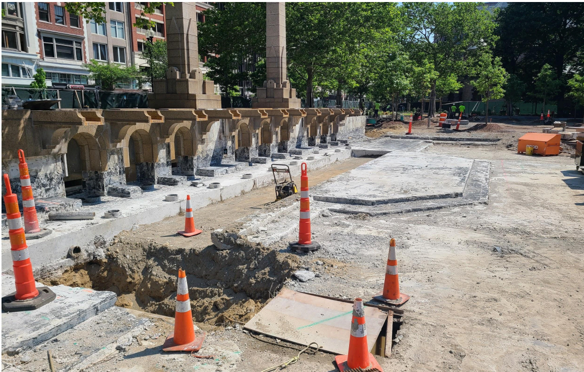
Excavation for new piping in the main fountain basin
