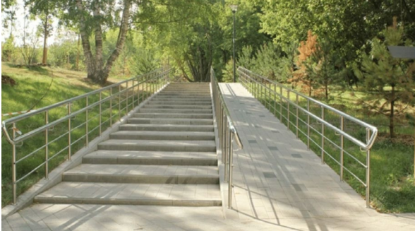
STAIR, RAMP & HANDRAIL PECEDENT IMAGE
