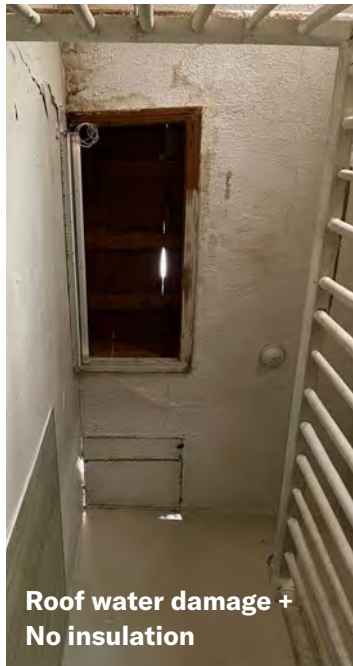
1st floor: damaged ceiling, water leakage
