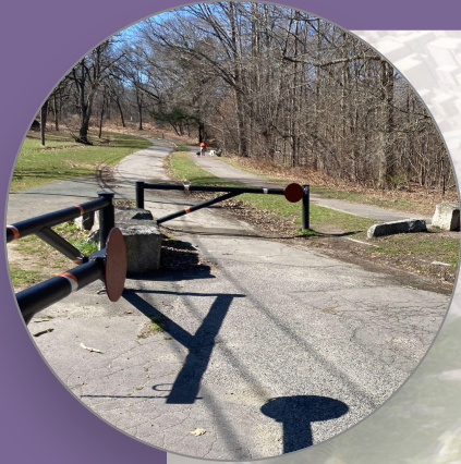
Example of Confusing Existing Circulation
