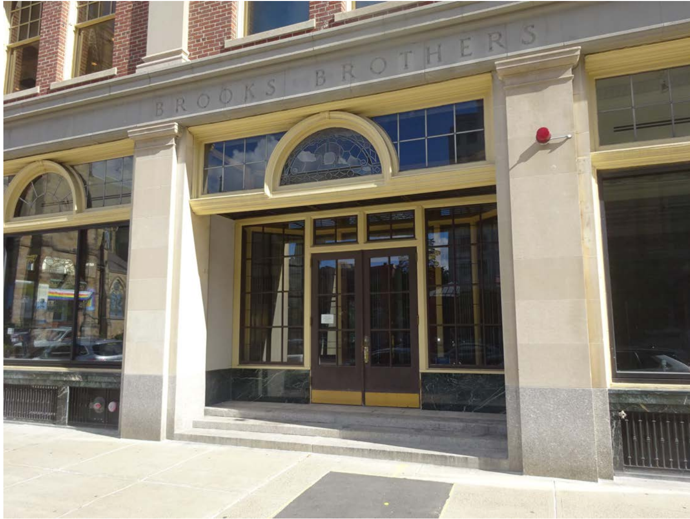
Existing Condition Photo
