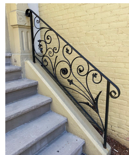
1615 Tremont St – East Railing
