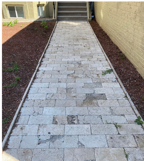
1615 Tremont St – Front Walkway
