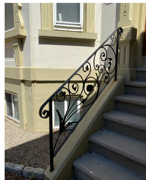
1615 Tremont St – West Railing
