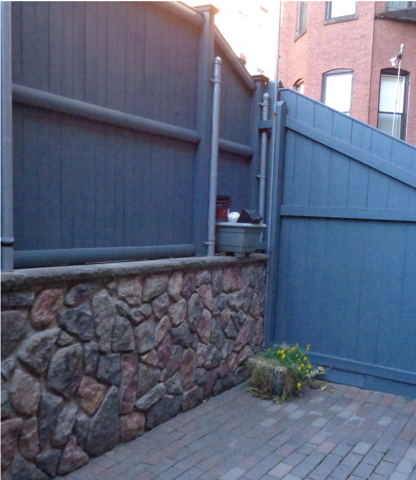
339 Marlborough Street Rear Garden Fence
