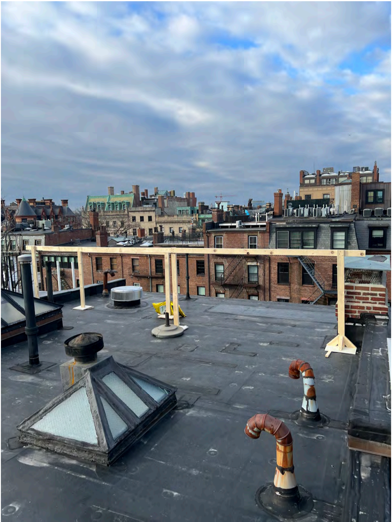
Mock up looking towards Alley 415
