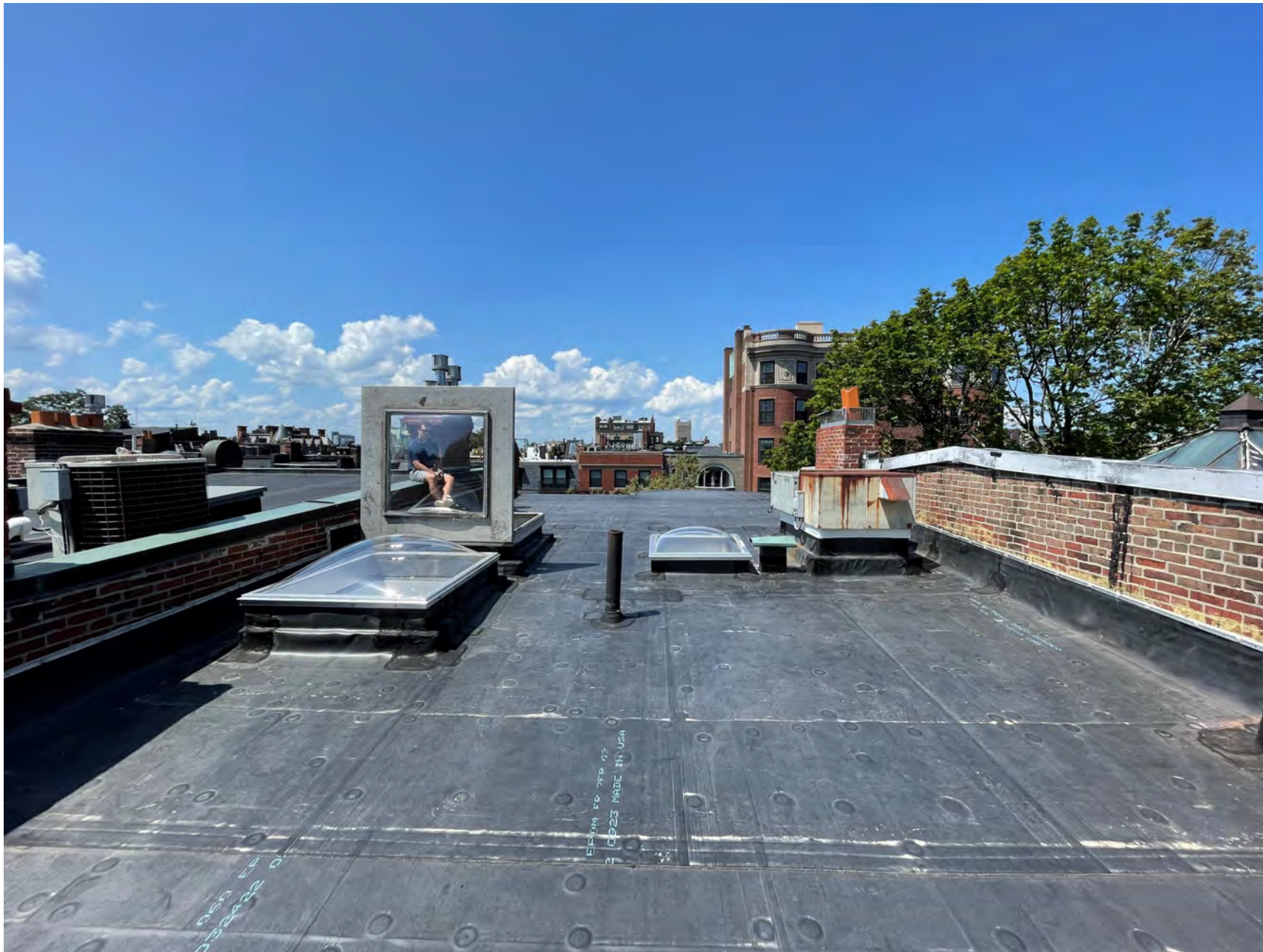
EXISTING ROOF LOOKING FROM REAR TO FRONT
