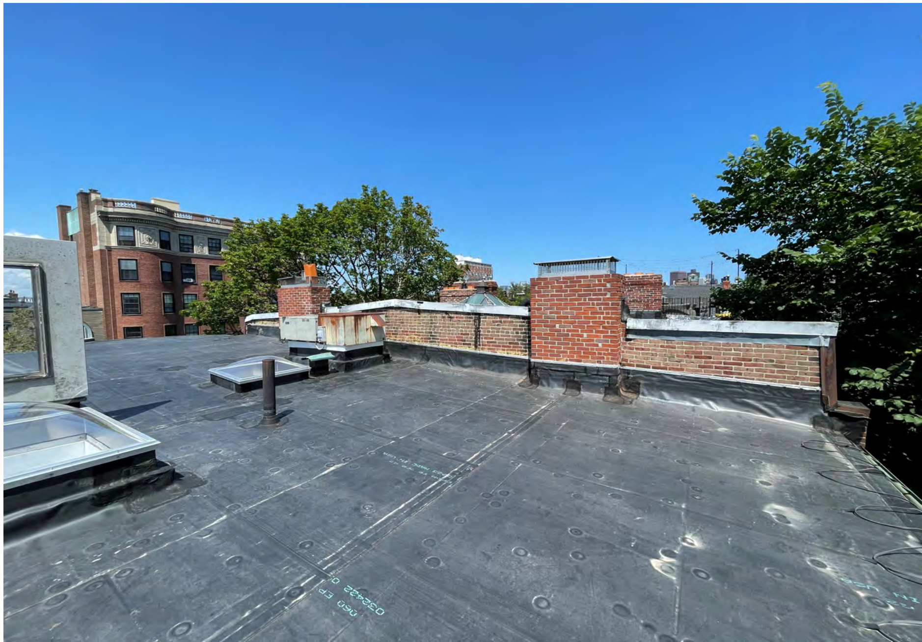
EXISTING ROOF LEFT SIDE PARAPET
