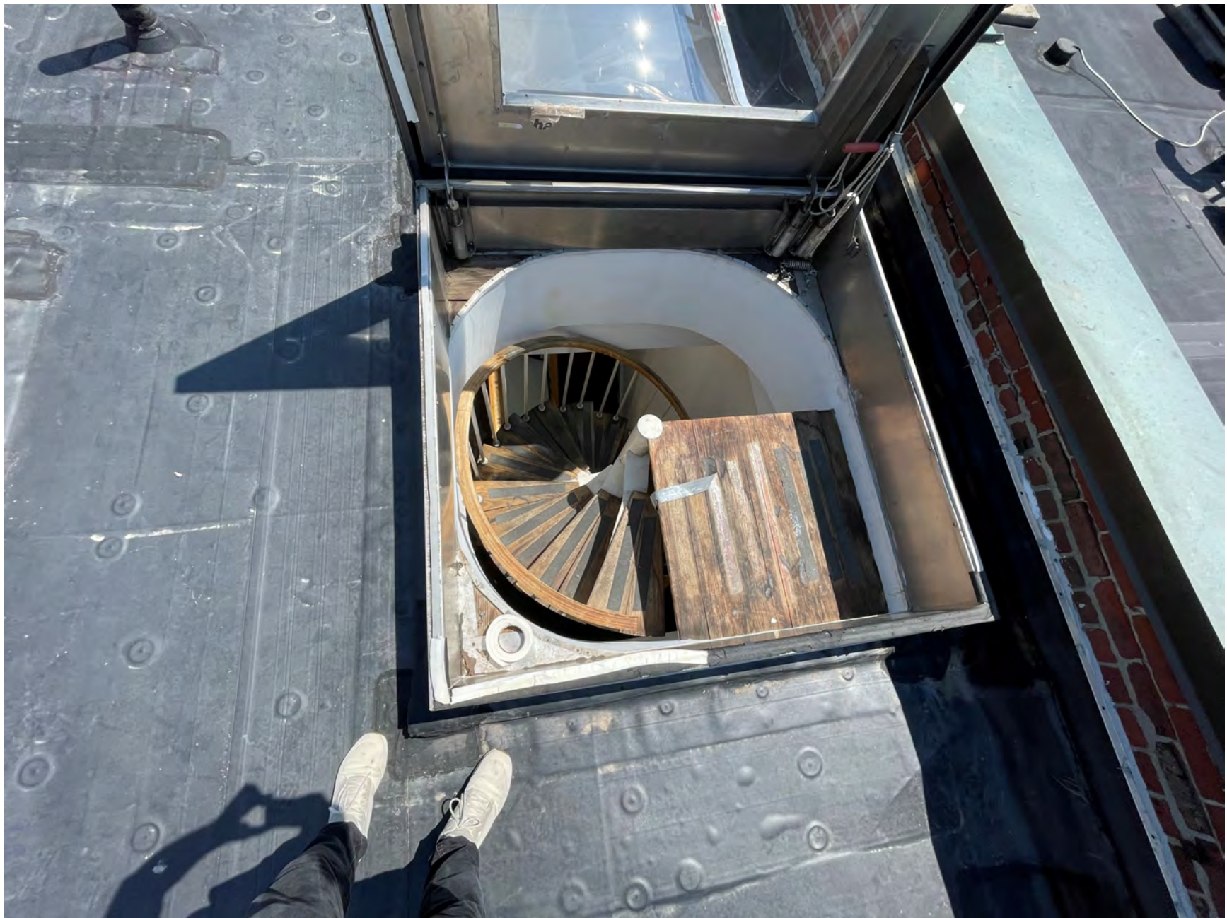
EXISTING ROOF HATCH AND STAIR
