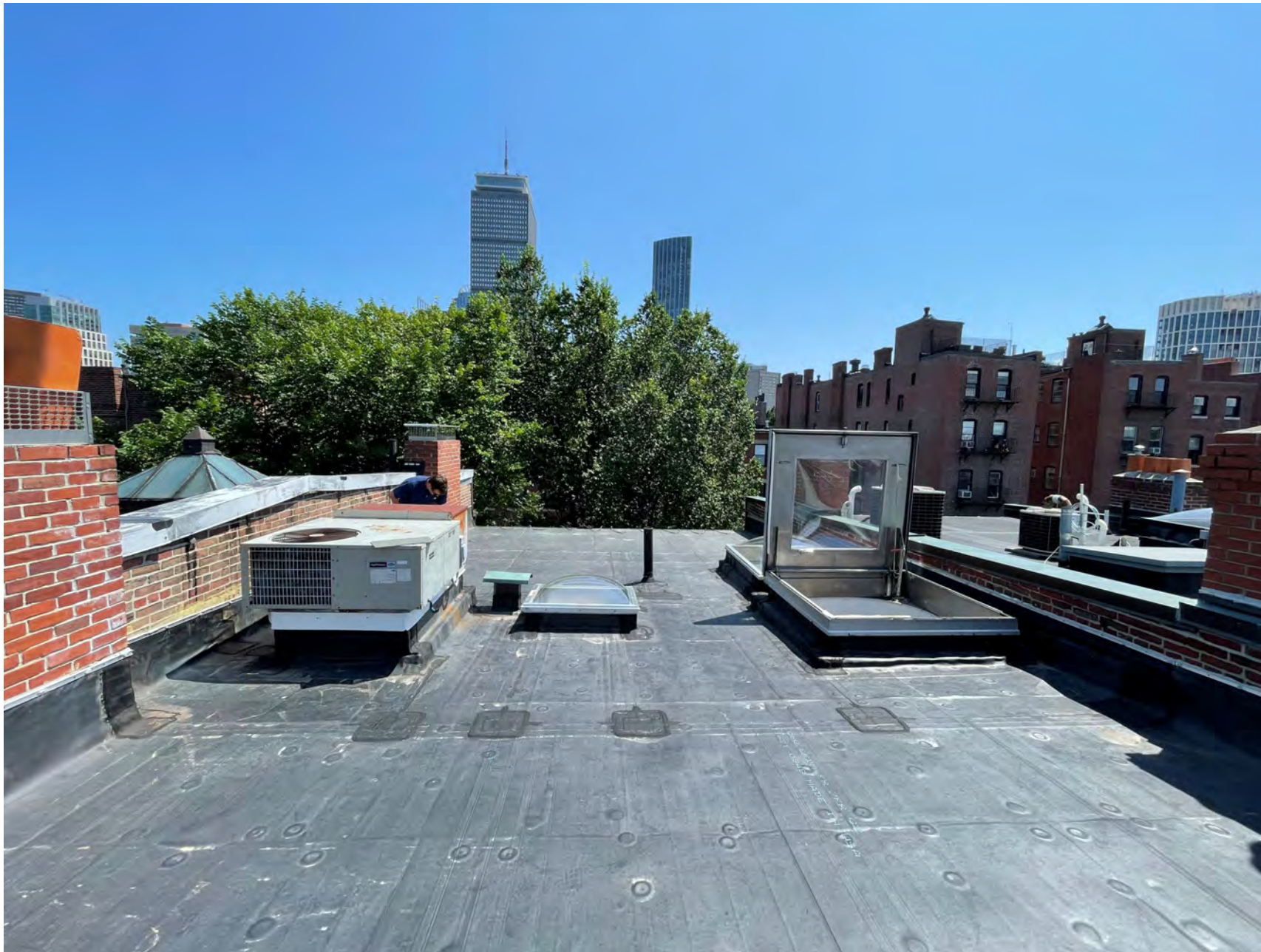
EXISTING ROOF LOOKING FROM FRONT TO REAR
