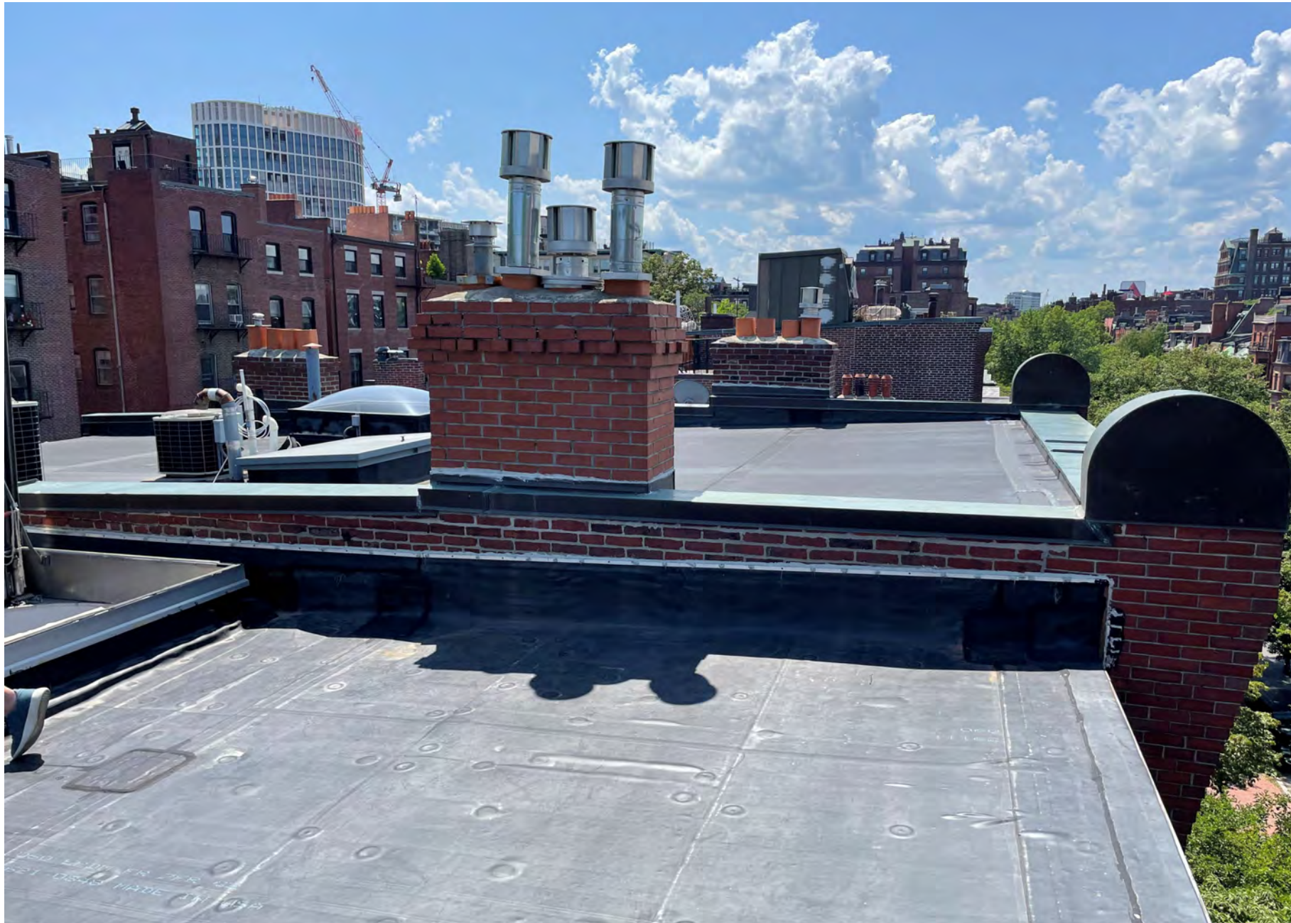
EXISTING ROOF RIGHT SIDE PARAPET FRONT
