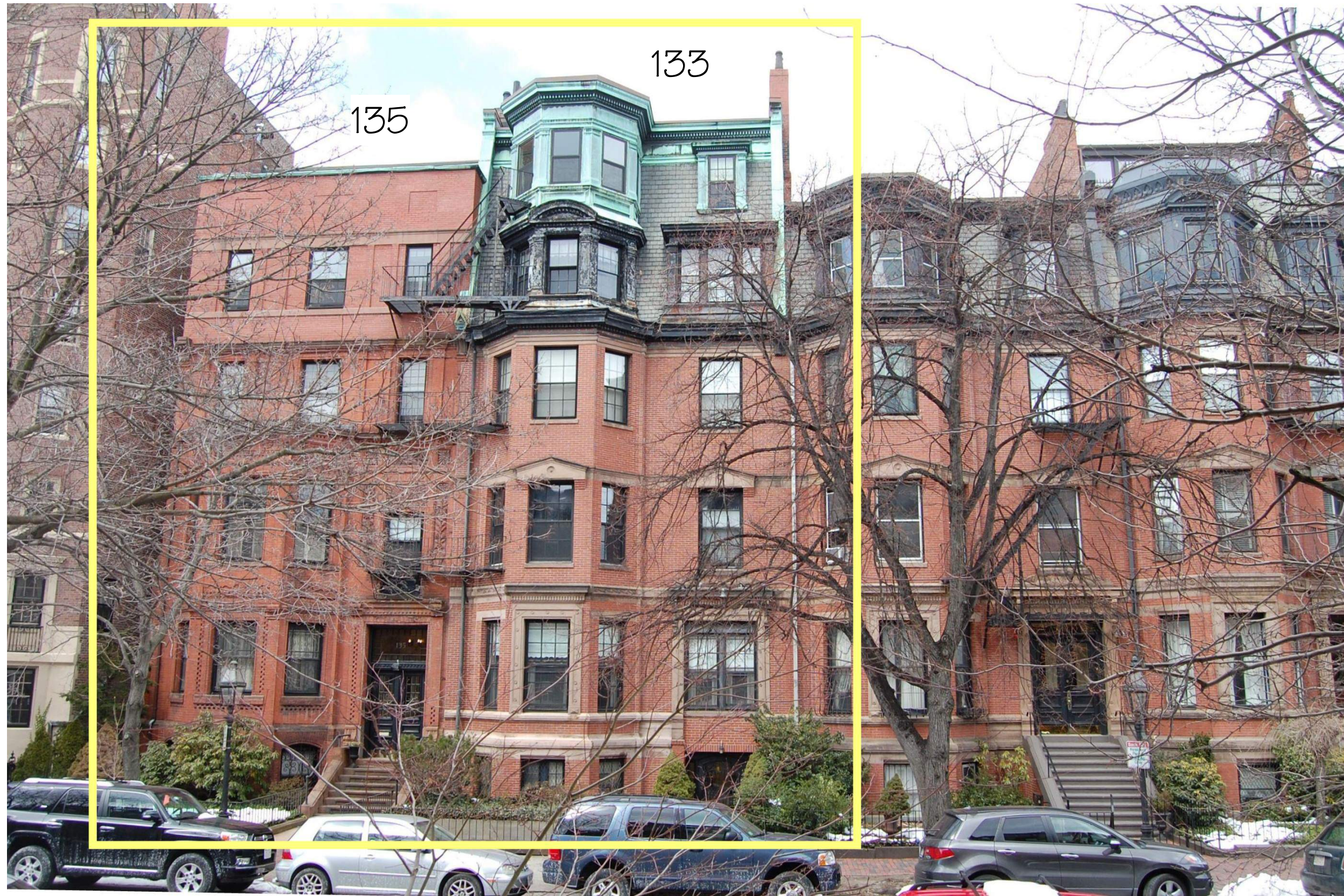
① Existing Photo (View #1)
