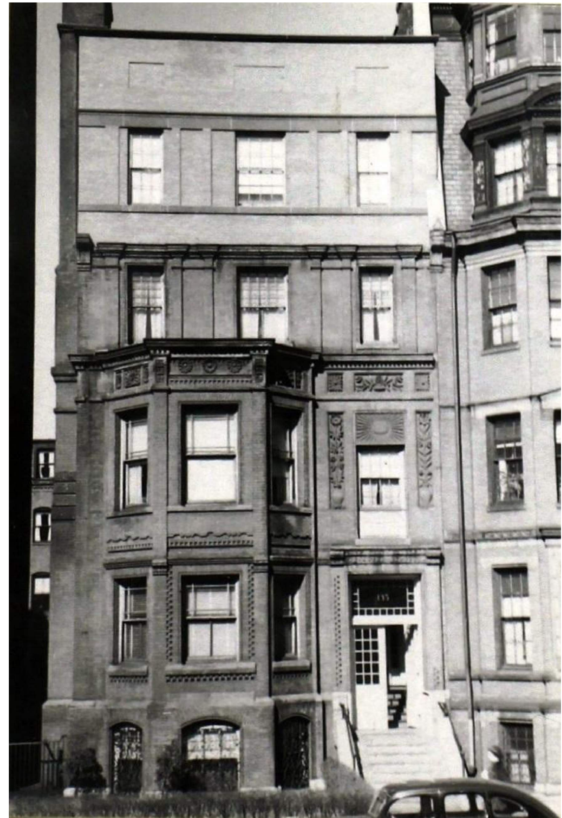
② 135 Marlborough Street (1942) After Renovation
