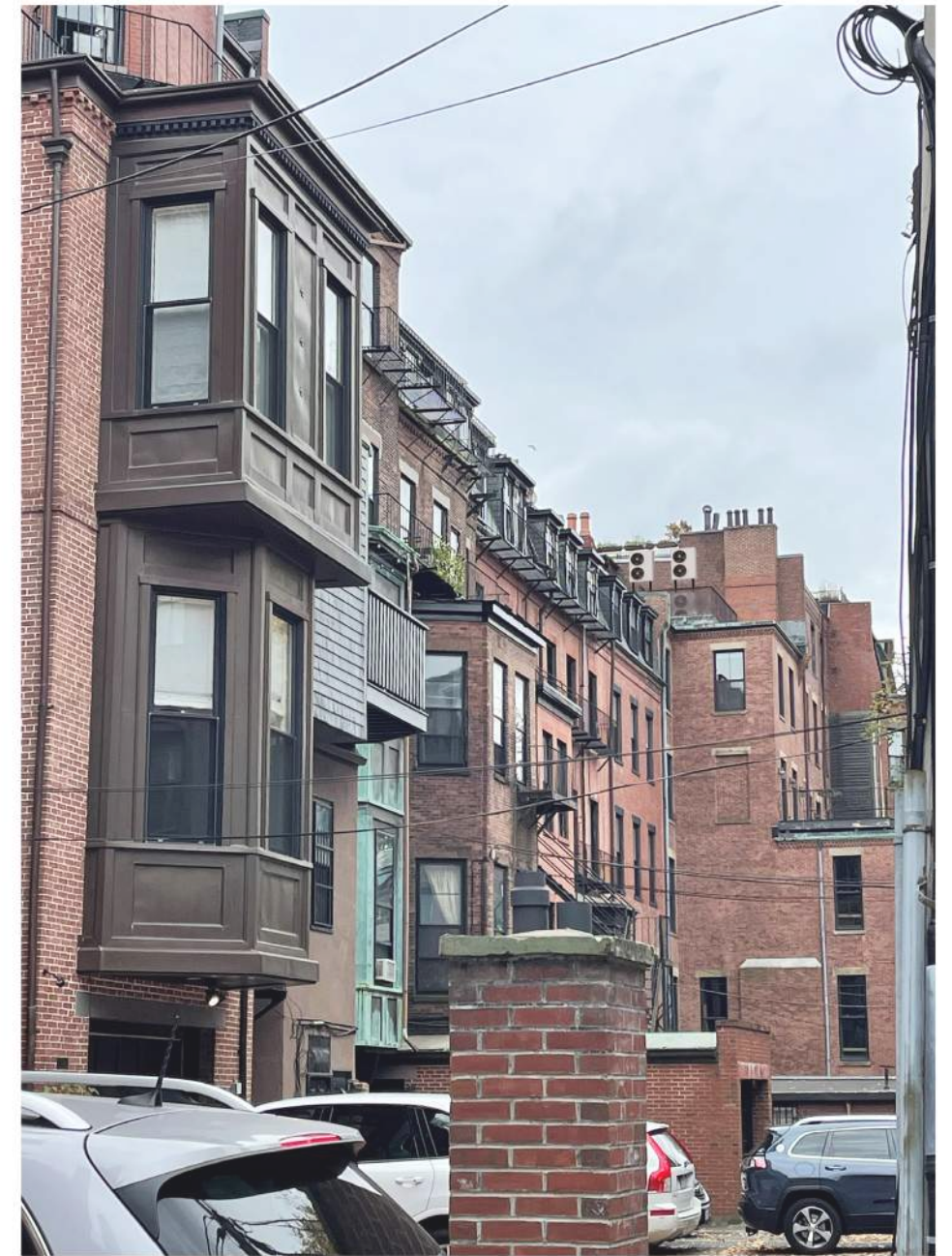
STACKED, NO ENCLOSURE
