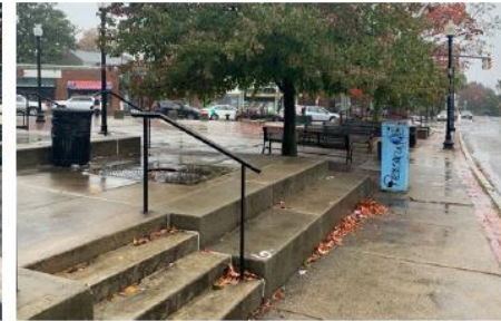
1.2 Complicated edge and access into park at Dudley St - multiple level steps, railing, seatwalls, ramp. Tree was removed and not replaced.
