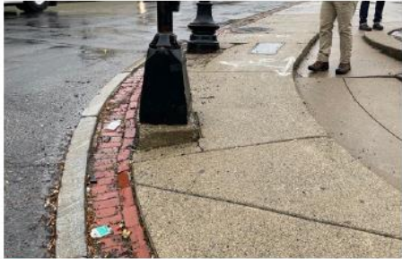
1.1 Cracking and heaving of concrete paving
