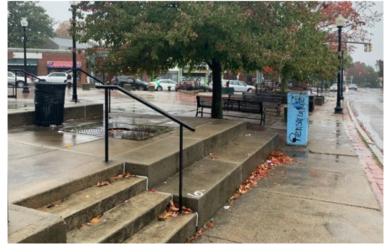
1.2 Complicated edge and access into park at Dudley St - multiple level steps, railing, seatwalls, ramp. Tree was removed and not replaced.
