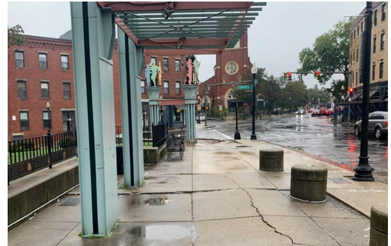
1.2 Bollards and shade structure do not contribute to bus stop and restrict site lines in park. Cracking and heaving of concrete paving. Outdated style.
