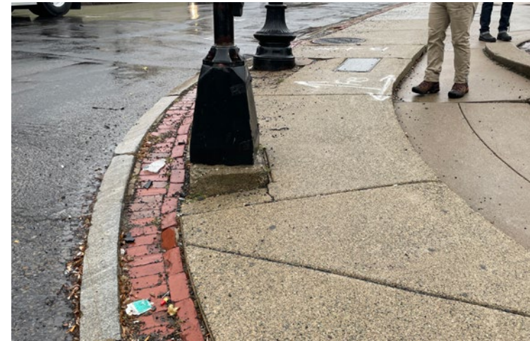
1.1 Cracking and heaving of concrete paving
