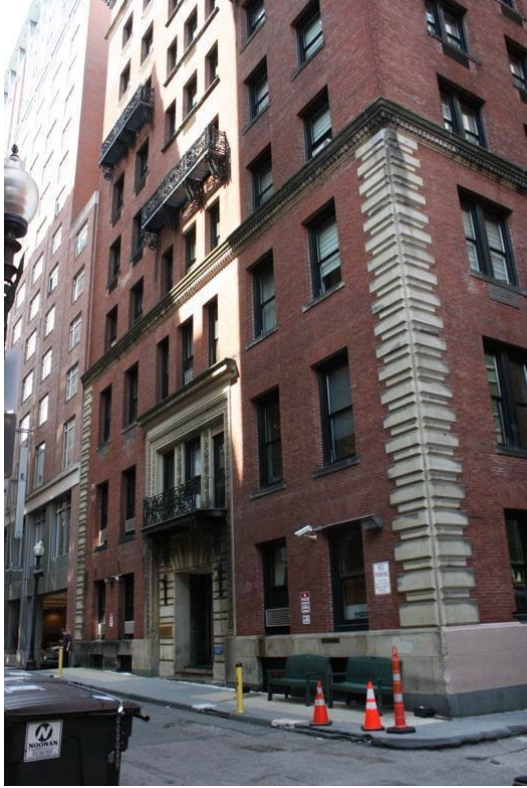
Figure 15. Parker House Annex; lower part of front façade (Bosworth Street). July 2020.
