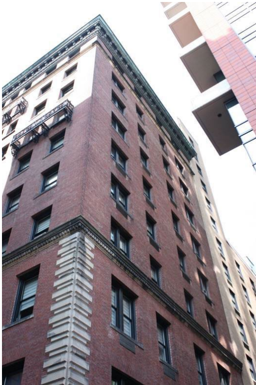
Figure 18. Parker House Annex; upper part of Chapman Place façade. July 2020.
