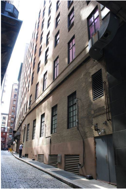
Figure 13. Chapman Place elevation, from School Street. July 2020.
