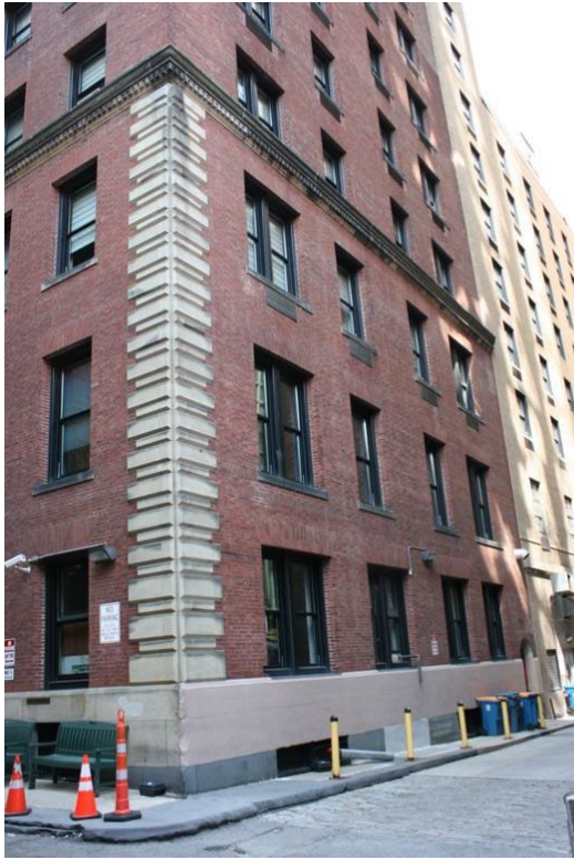
Figure 17. Parker House Annex; lower part of Chapman Place façade. July 2020.
