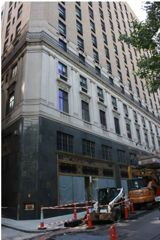
Figure 4. School Street (north) façade at Chapman Place. July 2020.
