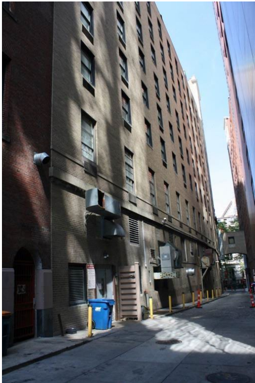
Figure 14. Chapman Place elevation, from Bosworth Street. July 2020.
