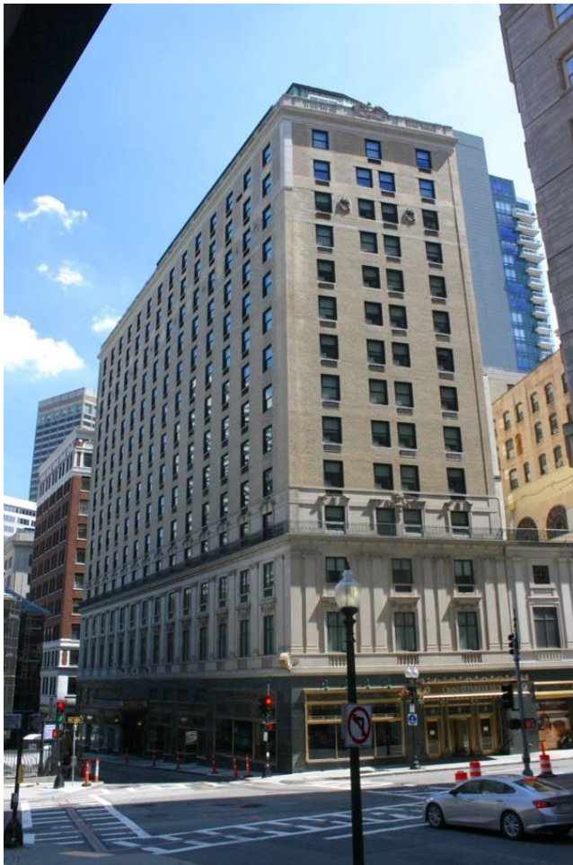
Figure 2. School Street (L) and Tremont Street (R) facades (main building). July 2020.
