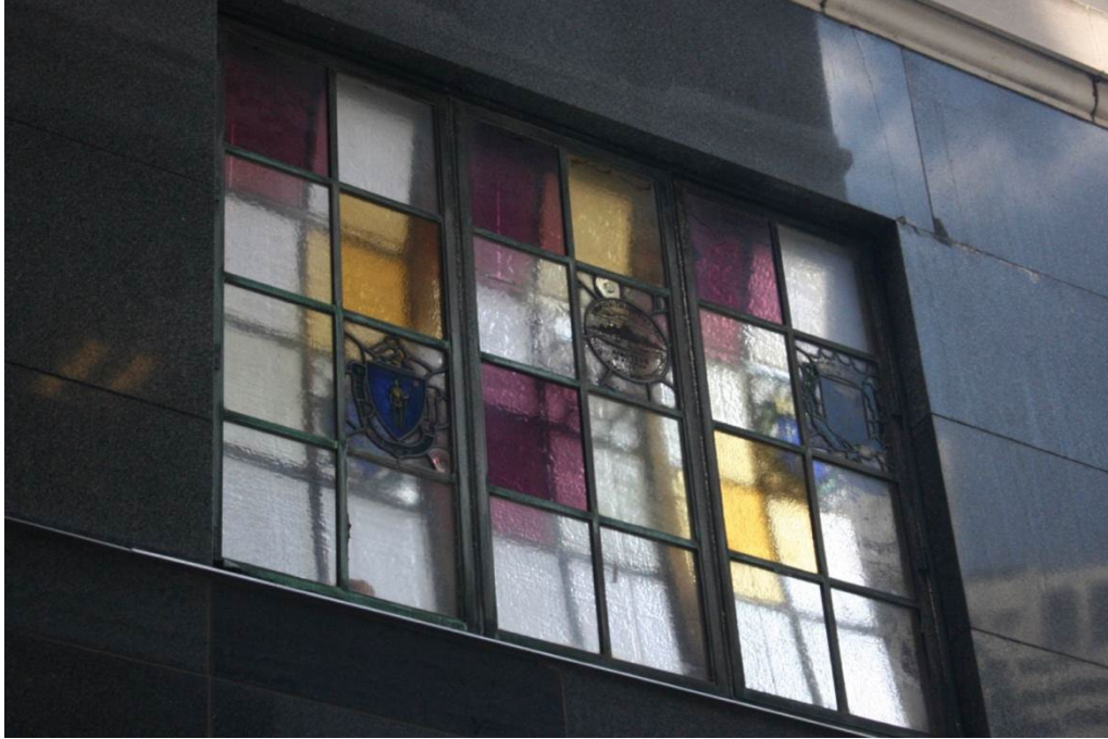
Figure 7. School Street façade; detail of stained and leaded glass above storefronts. July 2020.
