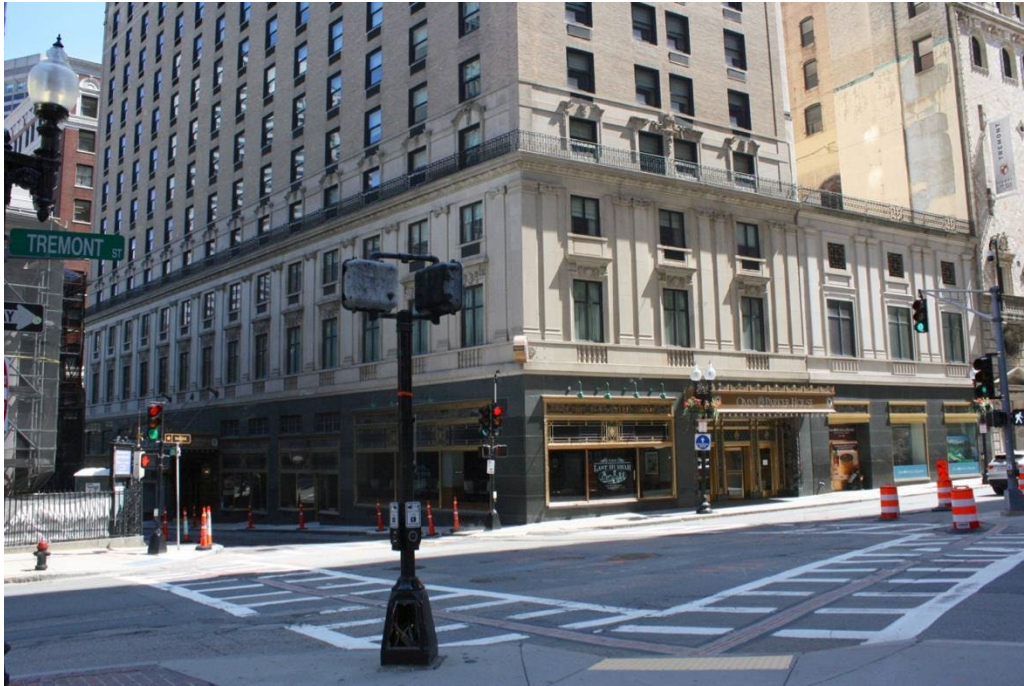
Figure 5. School and Tremont Street facades; storefronts and base. July 2020.
