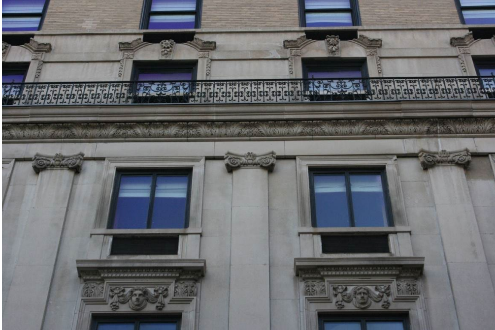
Figure 9. School Street façade; detail of trim at third, fourth, and fifth floors. July 2020.
