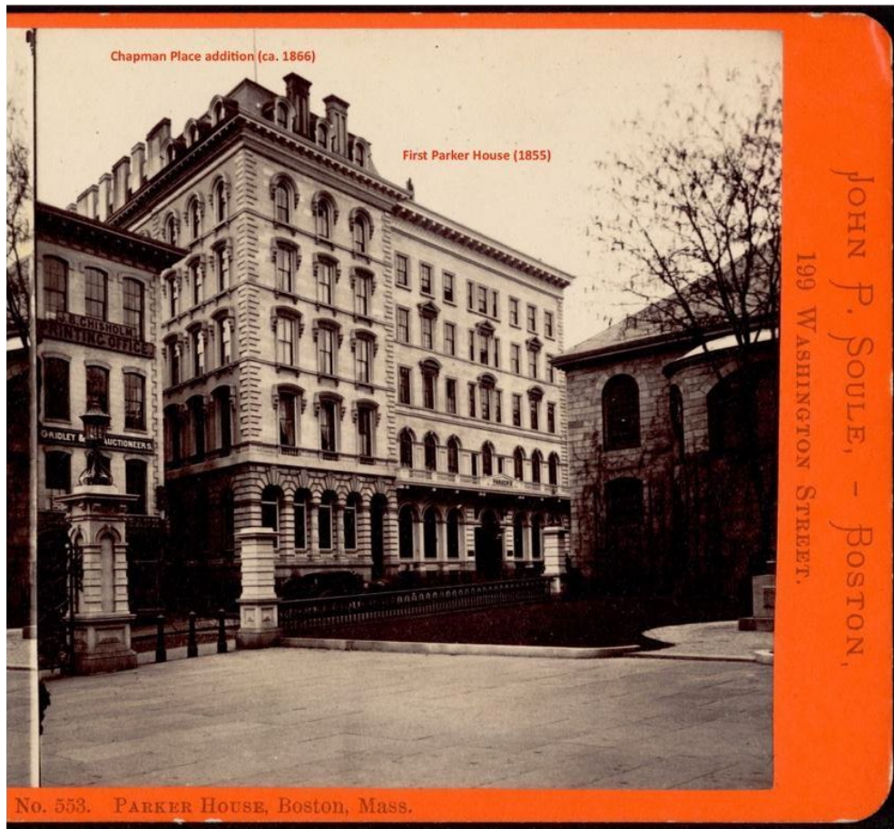
Historic Image 4. Parker House, ca. 1870s. View looking southwest on School Street from Old City Hall, showing Chapman Place addition (ca. 1866, left) and First Parker House (1855, right).
